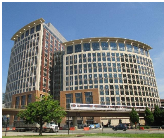
National Science Foundation Headquarters.
