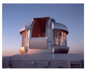
Gemini North dome/enclosure with setting sun (to left) lighting up the bottom half of the telescope through thermal vents (fully open). The observing slit is partially open, revealing the truss and top end of the telescope. *Credit: Neelon Crawford - Polar Fine Arts; courtesy of Gemini Observatory and NSF*
