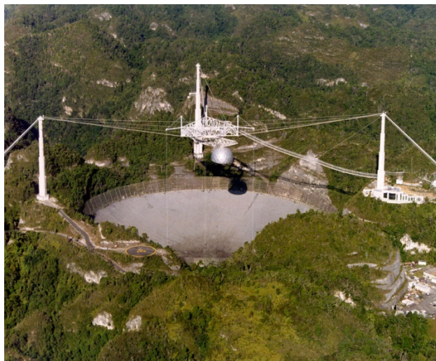
An aerial image of the Arecibo Radio Telescope in Puerto Rico. The platform suspension structure, including the Gregorian dome that houses the main suite of research instruments, is visible over the 305-meter primary reflector dish below. Credit: Arecibo Observatory/NSF.
