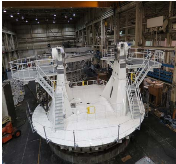
The mount base structure under construction. Credit: M. Warner, DKIST.
