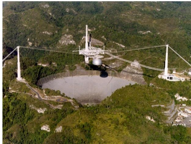
An aerial image of the Arecibo Radio Telescope in Puerto Rico. The platform suspension structure, including the Gregorian dome that houses the main suite of research instruments, is visible over the 305-meter primary reflector dish below. *Credit: Arecibo Observatory/NSF.*
