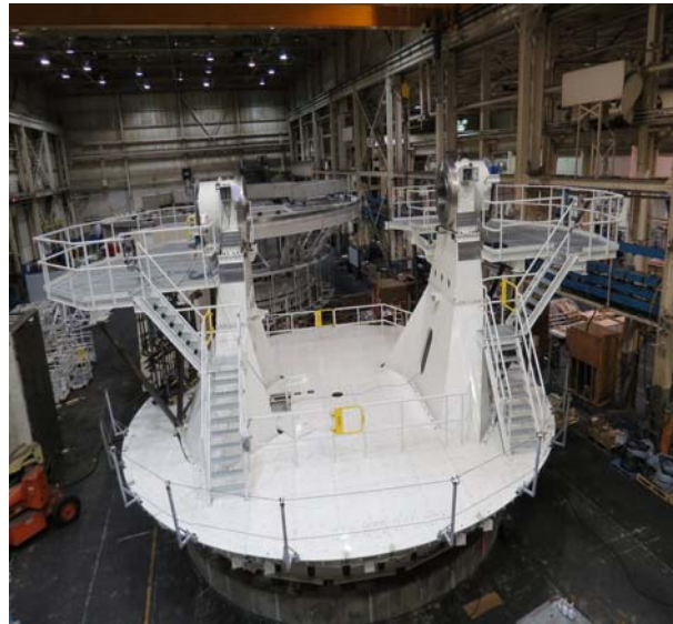
The mount base structure under construction. Credit: M. Warner, DKIST.
