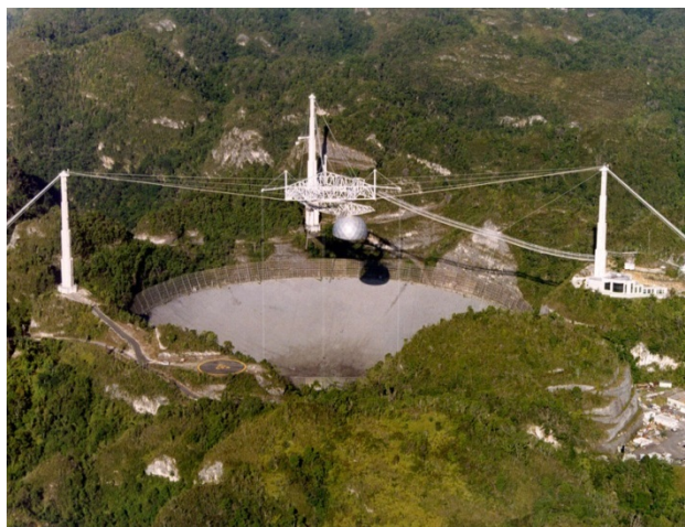
An aerial image of the Arecibo Radio Telescope in Puerto Rico. The platform suspension structure, including the Gregorian dome that houses the main suite of research instruments, is visible over the 305-meter primary reflector dish below. Credit: Arecibo Observatory/NSF.
