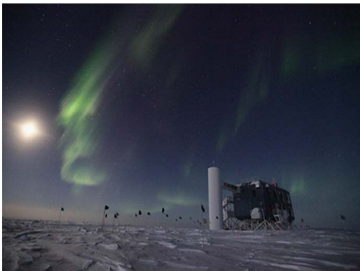
The IceCube project has transformed one cubic kilometer of natural Antarctic ice into a particle detector. The sensors keep watch for momentary flashes of blue light made by subatomic particles called muons; some are produced in collisions of neutrinos with atomic nuclei inside or near the detector. Since completion in 2010, the IceCube detector has been taking data in its final configuration with an up-time of well over 99 percent. IceCube detects one neutrino every 6 minutes in a background of 2700 cosmic ray muons per second. To handle the high rates, initial analysis of the data is performed by a cluster of computers housed in a two-story building placed on top of the array. The filtered data is sent over geostationary satellites to the IceCube Research Center at the University of Wisconsin. Credit: USAP Photo Library, Sven Lidstrom (sic), NSF.
