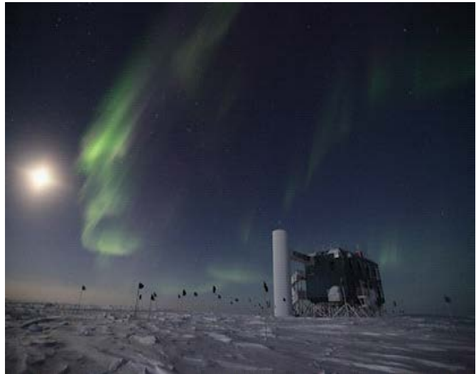
The IceCube project has transformed one cubic kilometer of natural Antarctic ice into a particle detector. The sensors keep watch for momentary flashes of blue light made by subatomic particles called muons; some are produced in collisions of neutrinos with atomic nuclei inside or near the detector. Since completion in 2010, the IceCube detector has been taking data in its final configuration with an uptime of well over 99 percent. IceCube detects one neutrino every 6 minutes in a background of 2700 cosmic ray muons per second. To handle the high data rates, initial analysis of the data is performed by a cluster of computers housed in a two-story building placed on top of the array. The filtered data is sent over geostationary satellites to the IceCube Research Center at the University of Wisconsin. Credit: USAP Photo Library, Sven Lidstrom (sic), NSF.
