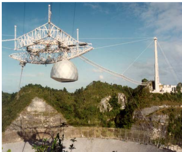
An image of the Arecibo Radio Telescope in Puerto Rico. The platform suspension structure, including the Gregorian dome that houses the main suite of research instruments, is visible over the 305-meter primary reflector dish below. Credit: Arecibo Observatory/NSF.
