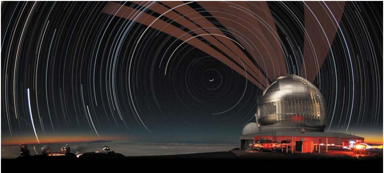
The Gemini North Telescope atop Mauna Kea in Hawaii. In this long-exposure photograph, the stars in the night sky appear as arcs due to the rotation of the earth. The reddish “beams” emanating from the top of the Gemini dome are produced by the laser used to support the observatory’s adaptive optics system. As the laser is tracked across the sky, following the target being observed, its narrow beam appears smudged in this time-lapse photograph. Credit: J. Pollard/Gemini Observatory
