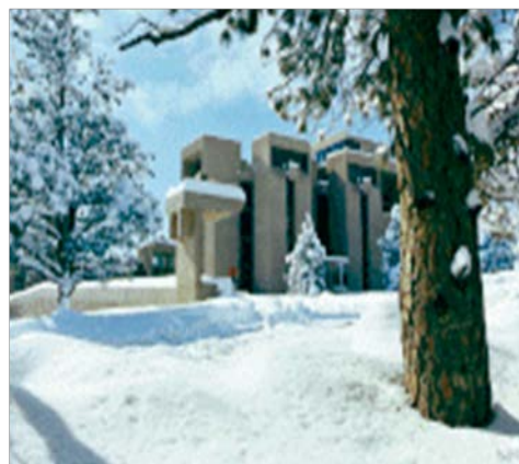
The Mesa Laboratory, designed by architect I.M. Pei, in Boulder, CO. Credit: NCAR.
