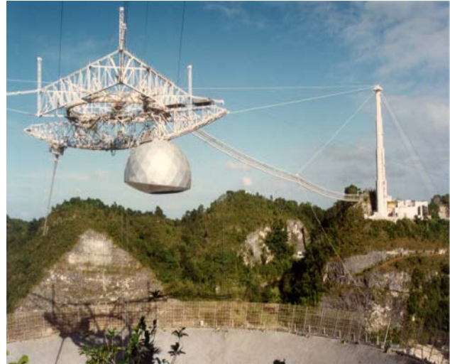
An image of the Arecibo Radio Telescope in Puerto Rico. The platform suspension structure, including the Gregorian dome that houses the main suite of research instruments, is visible over the 305-meter primary reflector dish below. Credit: Arecibo Observatory/NSF.
