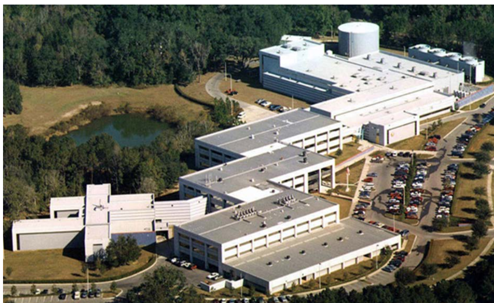
The National High Magnetic Field Laboratory, Tallahassee, Florida site. Credit: NHMFL
