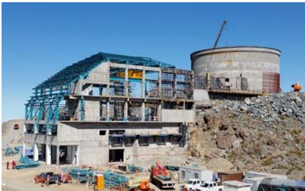
Construction status on Cerro Pachón, February 2017. Credit: LSST.
