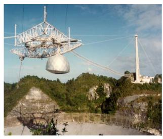
An image of the Arecibo Radio Telescope in Puerto Rico. The platform suspension structure, including the Gregorian dome that houses the main suite of research instruments, is visible over the 305-meter primary reflector dish below. *Credit: Arecibo Observatory/NSF*.
