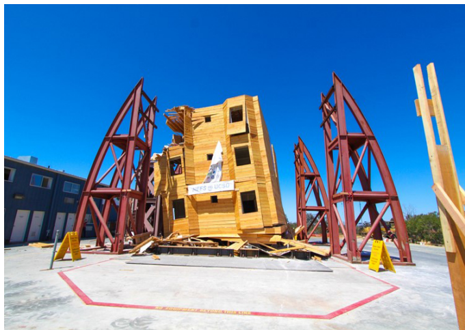
The above image displays the University of California, San Diego outdoor shake table, which allows large structures to be tested against seismic activity. Here, a wooden building shows damage after testing. Credit: UCSD/Jacobs School of Engineering.
