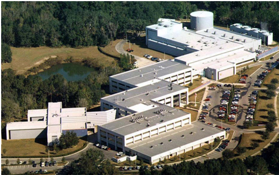
The National High Magnetic Field Laboratory, Tallahassee, Florida site. Credit: NHMFL
