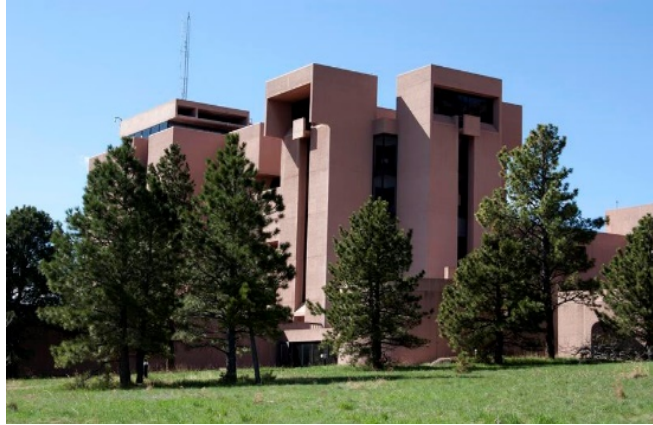
The NCAR Mesa Laboratory, designed by architect I.M. Pei, in Boulder, CO. Credit: UCAR.
