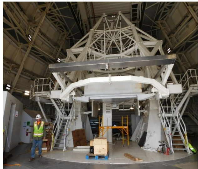
The Telescope Mount as of July 2017, showing two recently-completed Nasmyth platforms left and right of the main structure. Credit: P. Jeffers VSO/DKIST.
