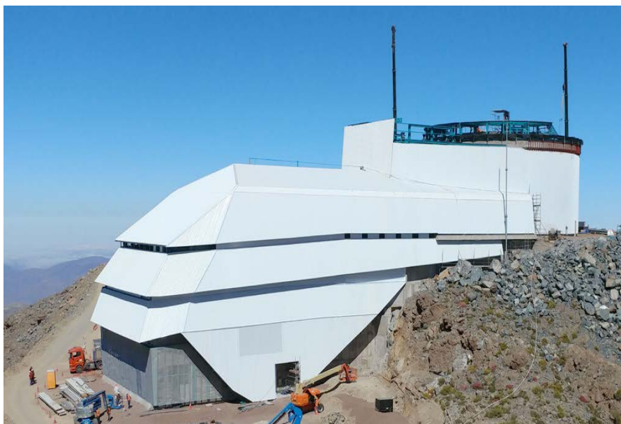
Construction status on Cerro Pachón, November 2017. Credit: LSST.
