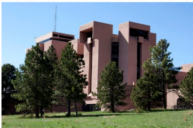
The NCAR Mesa Laboratory, designed by architect I.M. Pei, in Boulder, CO. Credit: UCAR.
