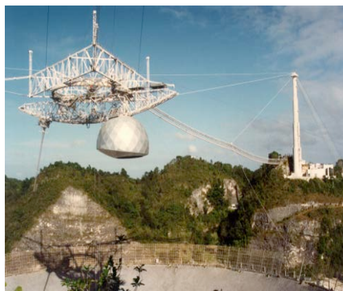
An image of the Arecibo Radio Telescope in Puerto Rico. The platform suspension structure, including the Gregorian dome that houses the main suite of research instruments, is visible over the 305-meter primary reflector dish below. The 96-foot line feed hanging to the left of the Gregorian dome was broken off during Hurricane Maria into several pieces, also damaging the dish below. Repairs are underway. Credit: Arecibo Observatory/NSF.
