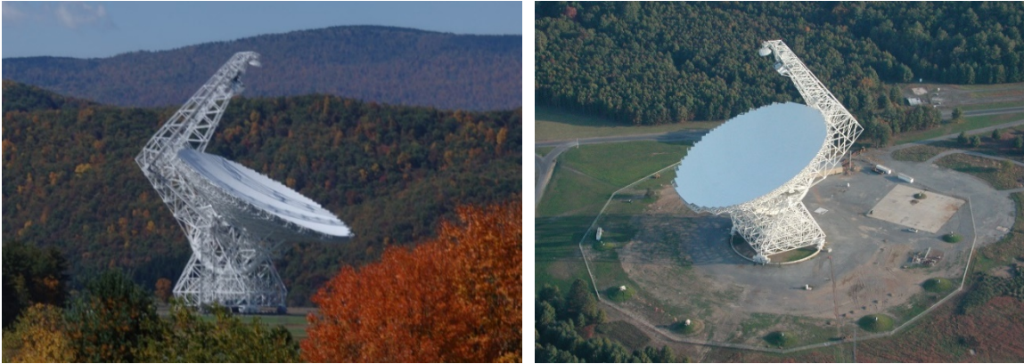
Views showing the Green Bank Telescope in the Fall (left) as well as the unblocked aperture and fully steerable structure (right). Credit: GBO/AUI.
