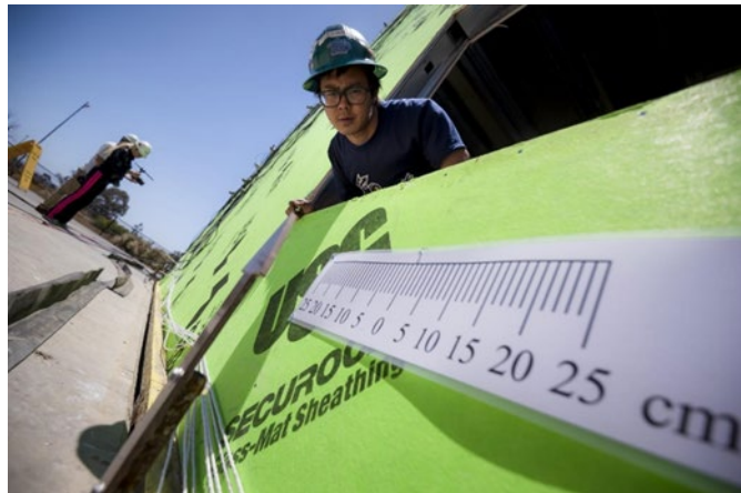
A graduate student inspects a six-story steel-framed building that is about to be tested on a shake table. Credit: UC San Diego
