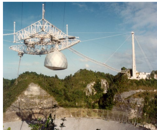
An image of the Arecibo Radio Telescope in Puerto Rico. The platform suspension structure, including the Gregorian dome that houses the main suite of research instruments, is visible over the 305-meter primary reflector dish below. The 96-foot line feed hanging to the left of the Gregorian dome was broken off during Hurricane Maria into several pieces, also damaging the dish below. Repairs are underway. Credit: Arecibo Observatory/NSF.
