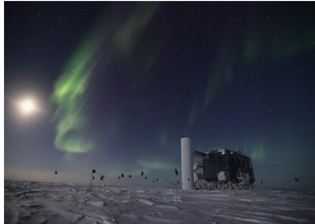
The IceCube Laboratory building at South Pole where all data-collecting computer servers are located. Credit: USAP Photo Library, Sven Lidstrom, NSF.
