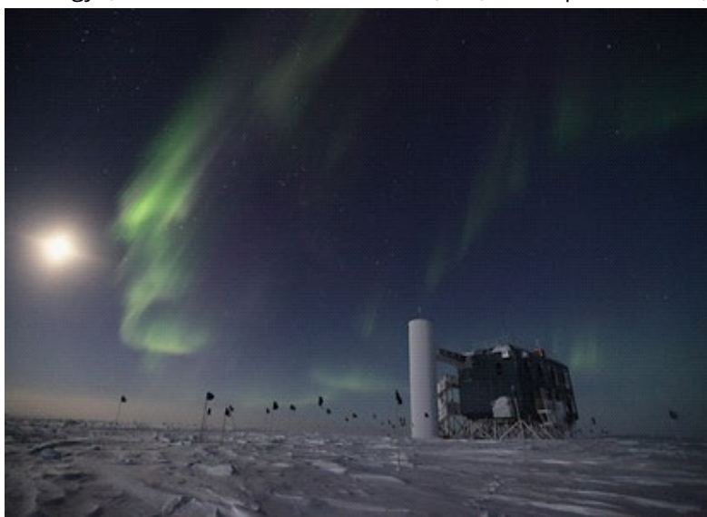
The IceCube Laboratory building at South Pole where all data-collecting computer servers are located. Credit: USAP Photo Library, Sven Lidstrom, NSF.
