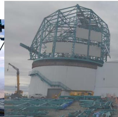
Summit 80 Ton lift completed. Dome panel installation begins
