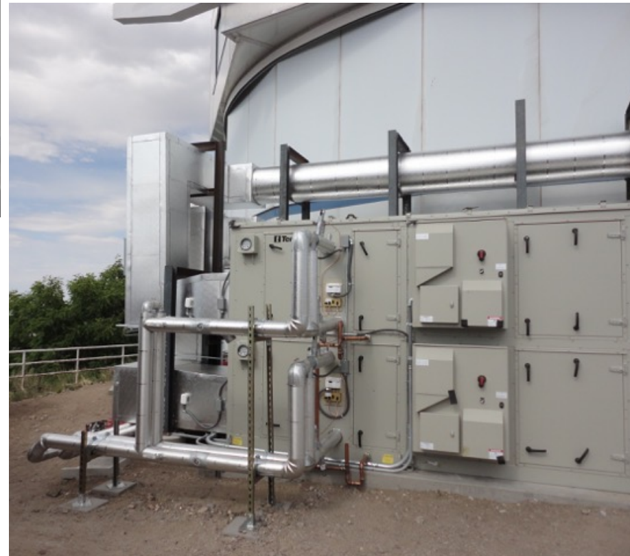
Extensive new HVAC system for stable environmental control
