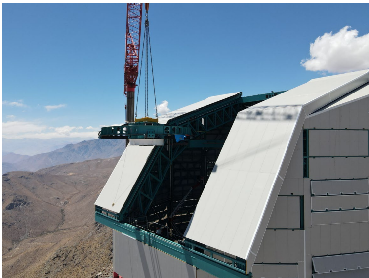
Telescope mount top end lifted into dome (Mar. 2021)
