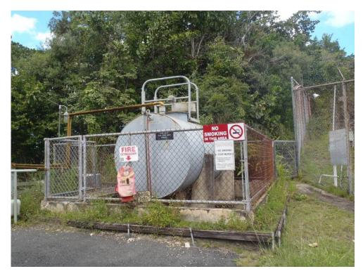
Photo 54: 2,000-gallon diesel tank for emergency generator facing west.
