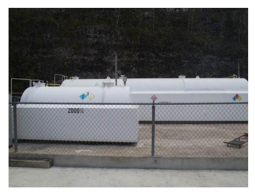
Photo 53: 2,000-gallon gasoline aboveground storage tank and 12,000-gallon diesel aboveground storage tank facing south.
