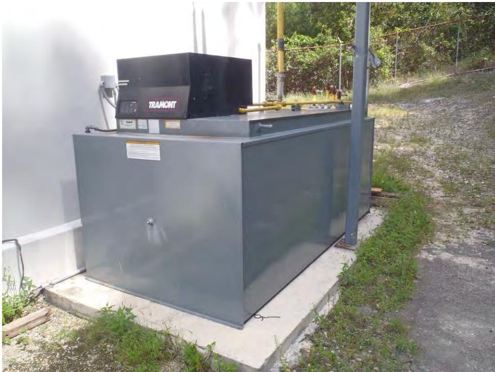
*Photo 52: 1,000-gallon day tank for generator at Building #80.*
