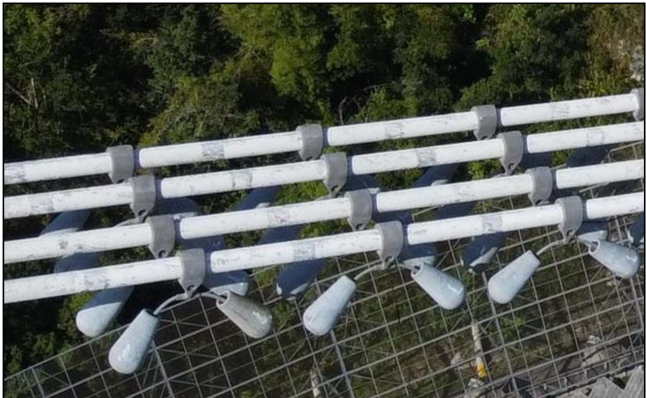
Figure 10: Stockbridge dampers on original M4 cables (photo: NAIC Arecibo Observatory, a facility of the NSF).
