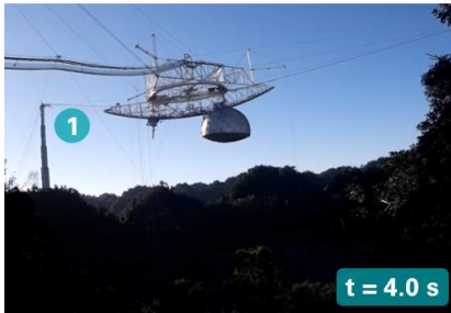
Figure 19: Telescope collapse sequence, looking south. (Still images of collapse video by NAIC Arecibo Observatory, a facility of the NSF. Intermediate still images are in provided Appendix E.)
