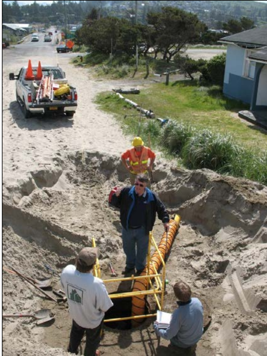
Figure 2-19. View looking east from the existing BMH
