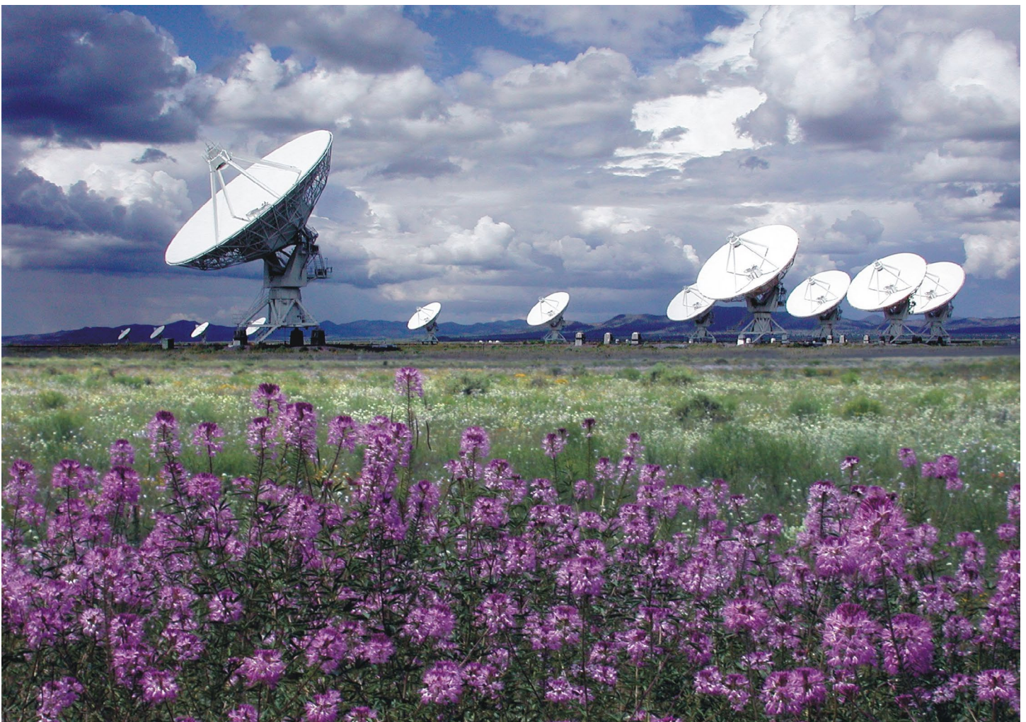
The NSF NRAO Very Large Array (NSF VLA) telescope is located on the Plains of San Agustin, about 80 kilometers west of the Array Operations Center in Socorro, New Mexico. The VLA is composed of 27 individual antennas arranged in a "Y" pattern. Four times each year, the VLA antennas are moved into new configurations by a transporter that moves along dual sets of railroad tracks. In their closest configuration (about 1 kilometer wide) the VLA is able to image large portions of the sky. In its largest configuration (about 36 kilometers wide) the VLA is able to hone in on the fine details of astronomical objects. Image credit: NRAO/AUI and photographer Kelly Gatlin; digital composite, Patricia Smiley
