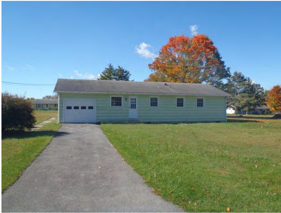
Photo 39: House # 4 facing southwest.
