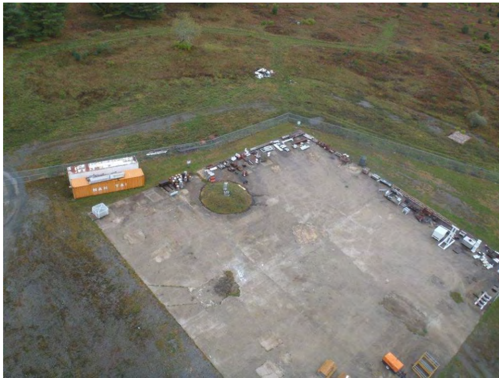
Photo 18: GBT storage yard facing west.
