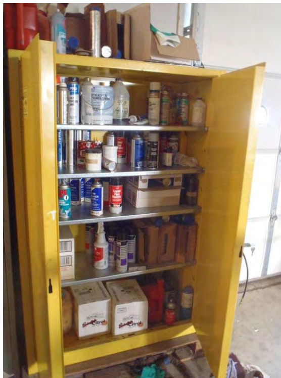
Photo 87: Flammable locker in Works building.
