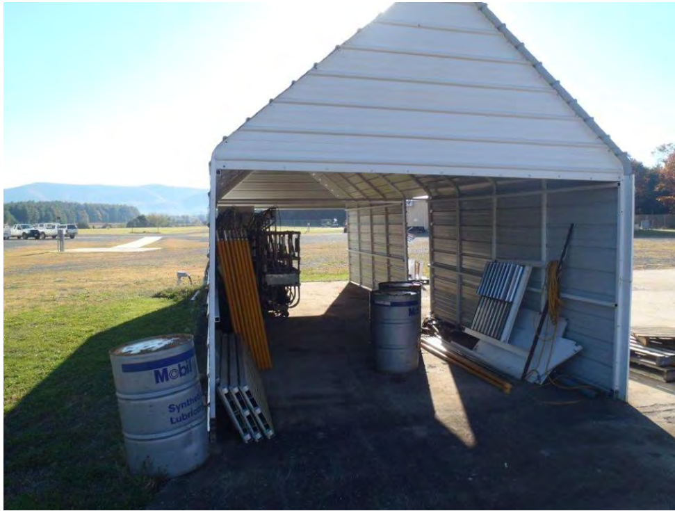
Photo 19: GBT storage yard shed facing east.
