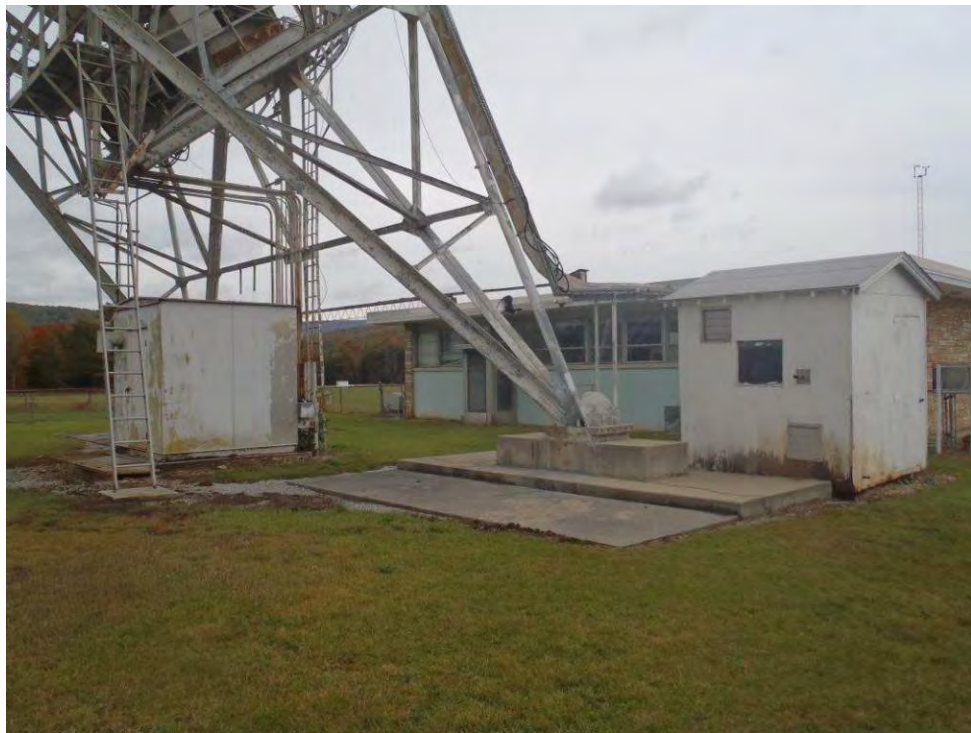
Photo 22: Shed at 85-1 facing northeast.
