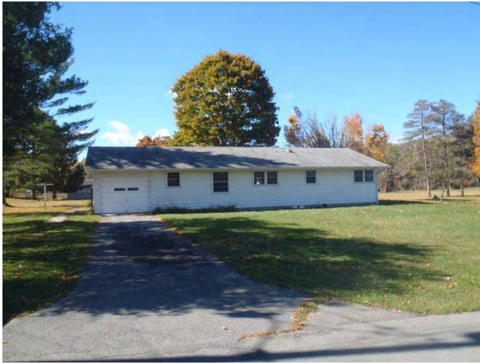
Photo 43: House #8 facing southwest.
