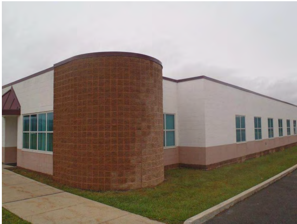
Photo 34: Bunk house facing north.
