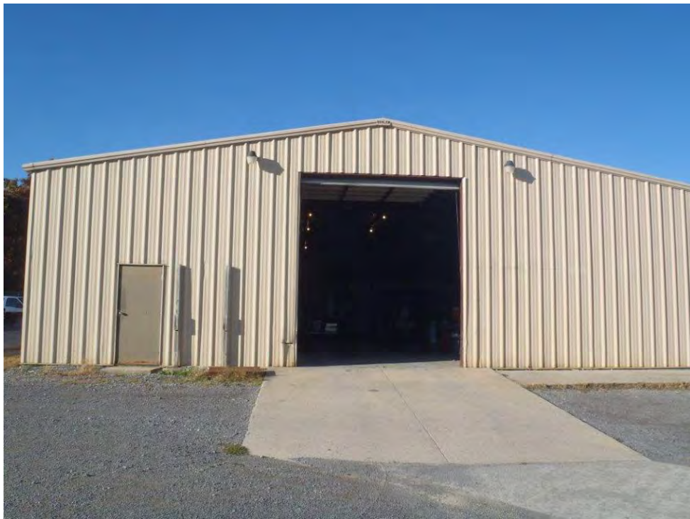
Photo 16: GBT storage building facing west.
