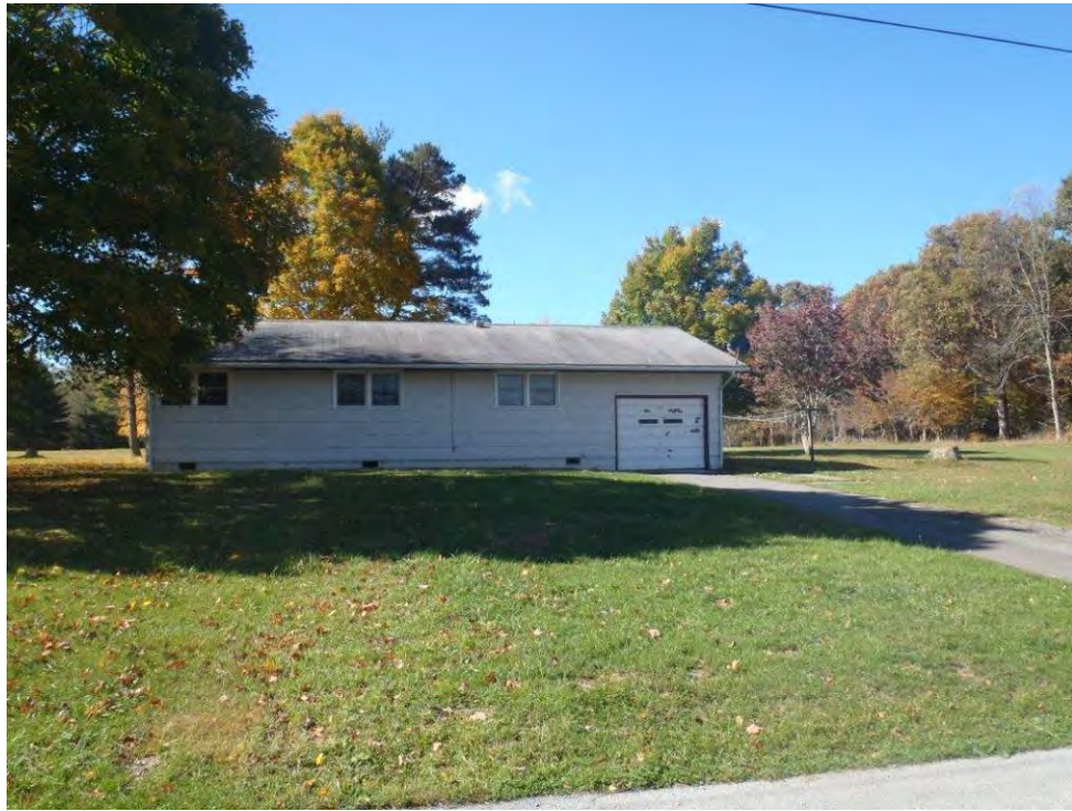
Photo 45: House #10 facing southwest.
