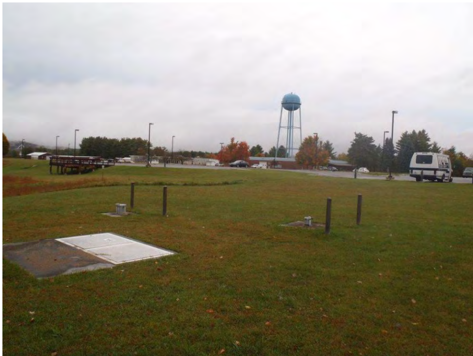
Photo 72: Drinking water wells facing north.
