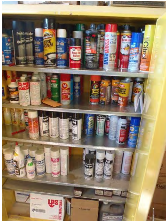
Photo 90: Flammable locker in Works building.
