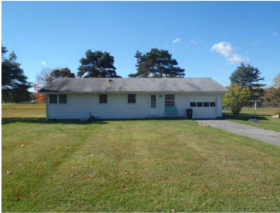
Photo 37: House #2 facing southwest.
