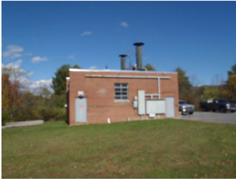
Photo 33: Paint booth facing north.
