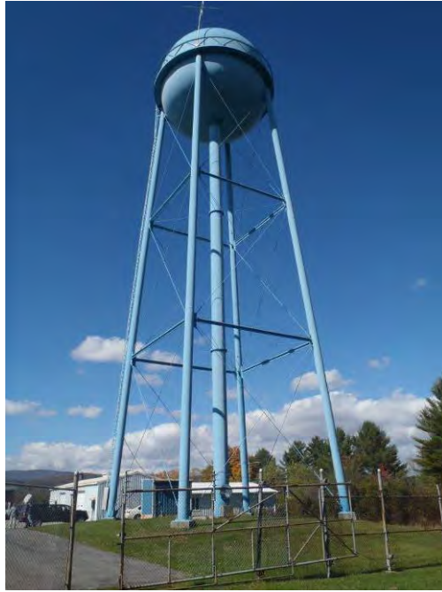
Photo 73: 100,000-gallon water tower facing northwest.
