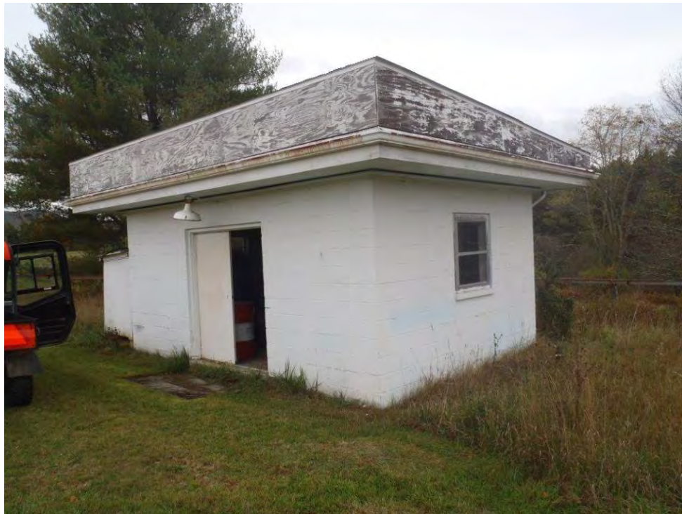
Photo 66: Sheds southwest of 85-1.
