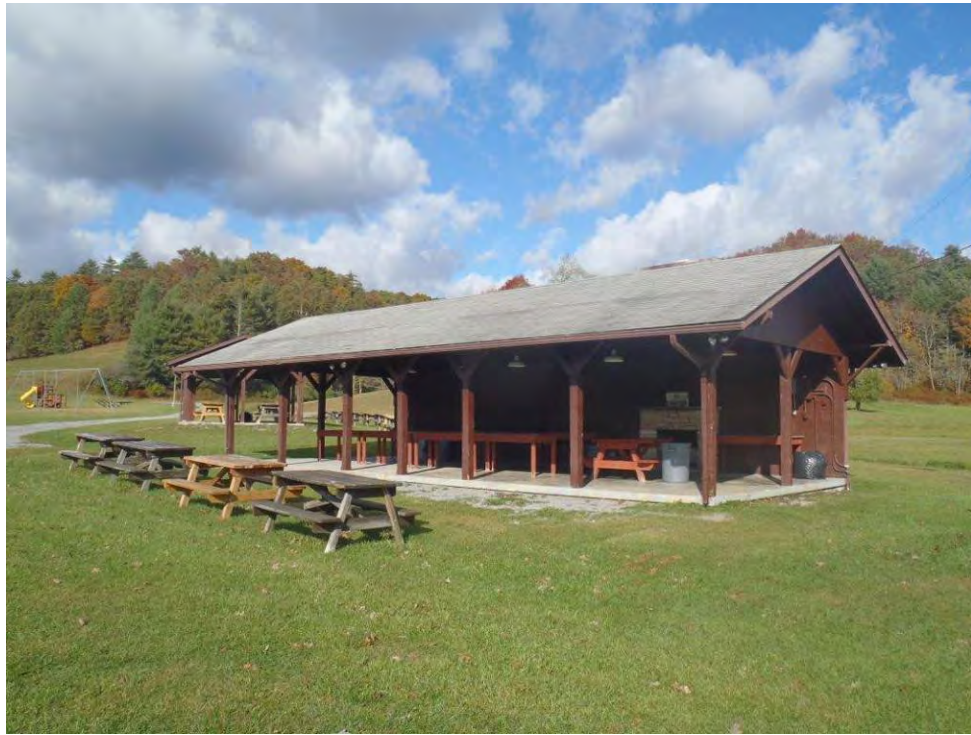
Photo 61: Pavilion facing north.
