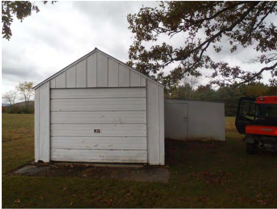
Photo 65: Sheds east of 85-1.
