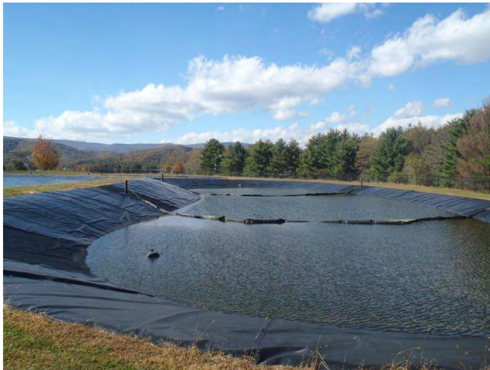
Photo 74: Wastewater treatment ponds facing west.
