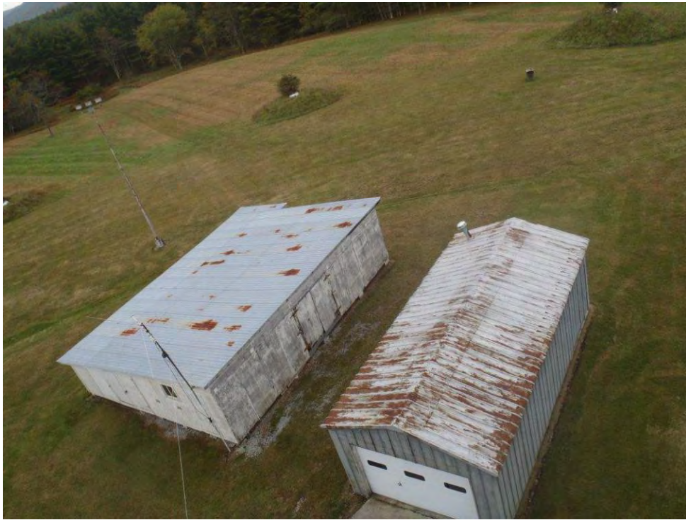
Photo 69: 140-telescope sheds facing east.
