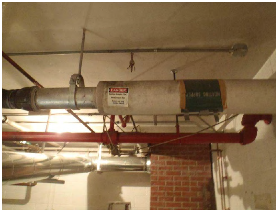
Photo 103: Encapsulated ACM at Jansky Laboratory.
