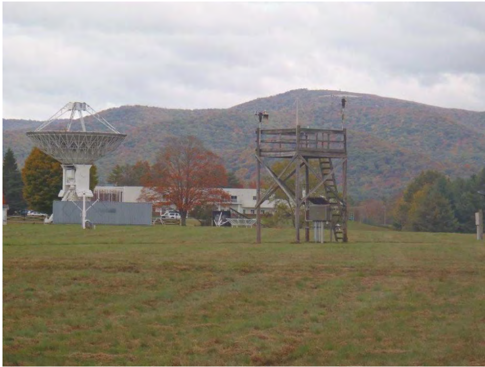
Photo 67: Weather station facing north.
