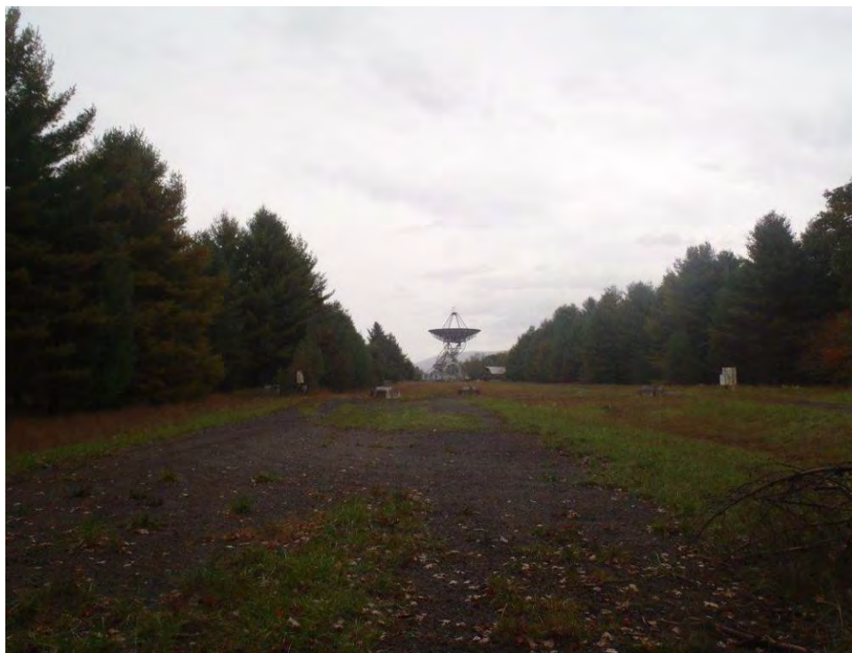
Photo 8: 85-2 interferometer facing northeast.
