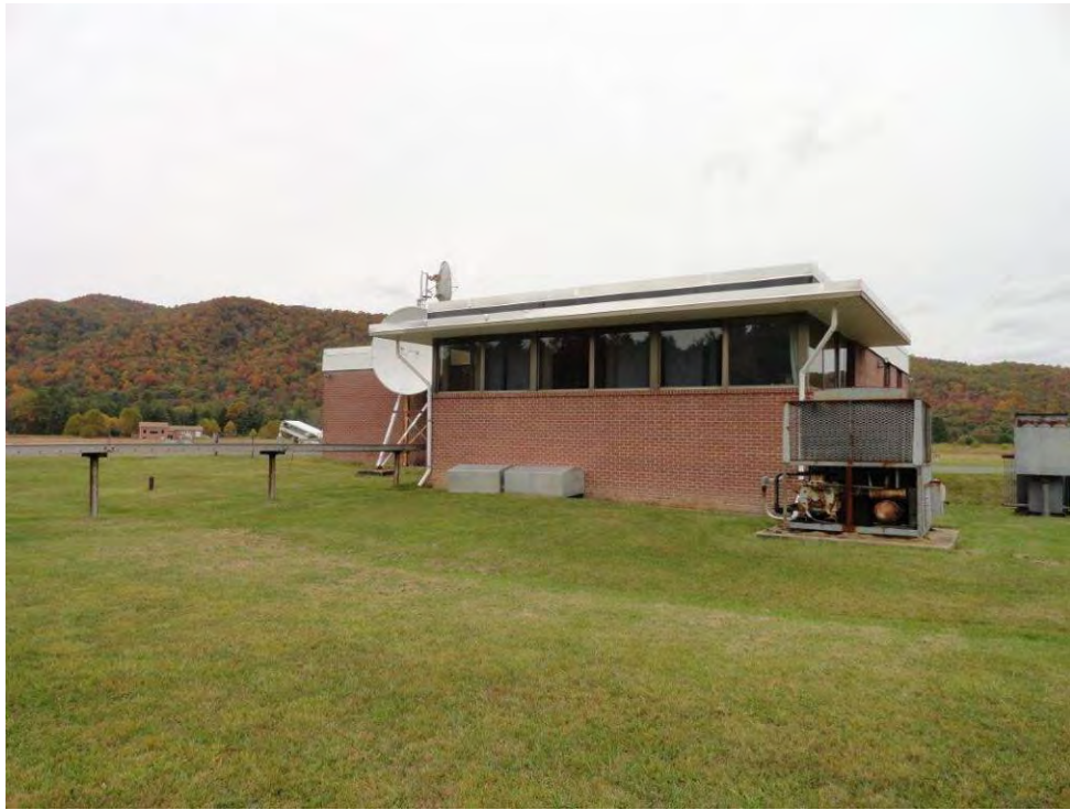
Photo 11: Former interferometer control building facing north.
