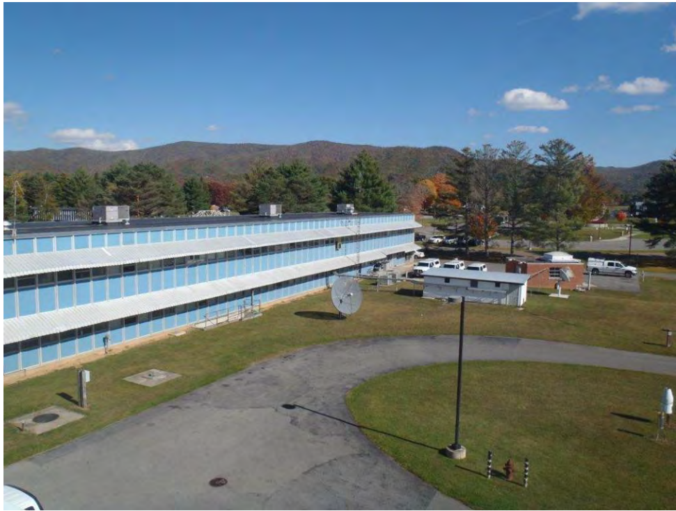
Photo 27: Jansky Laboratory facing northeast.
