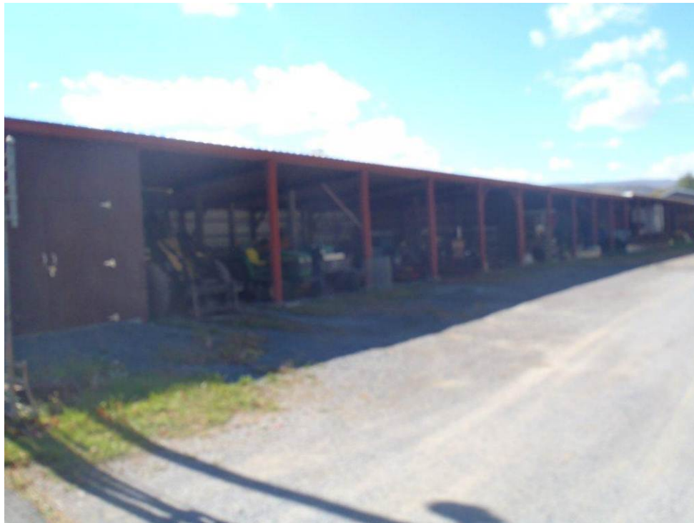
Photo 30: Covered storage at works area facing west.
