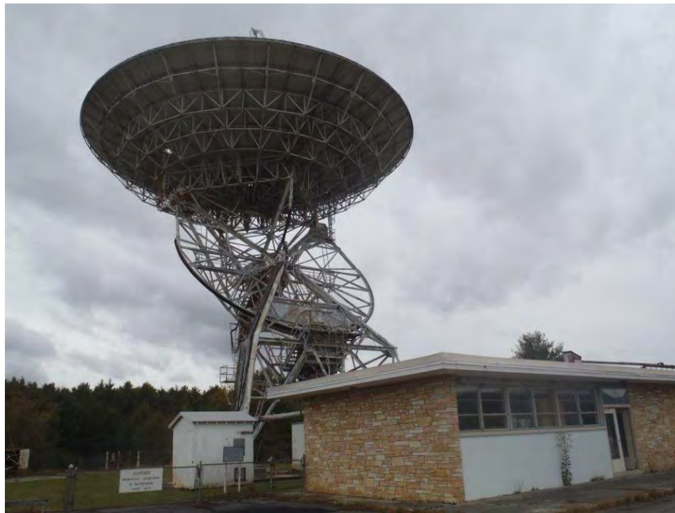
Photo 7: 85-1 interferometer facing south.
