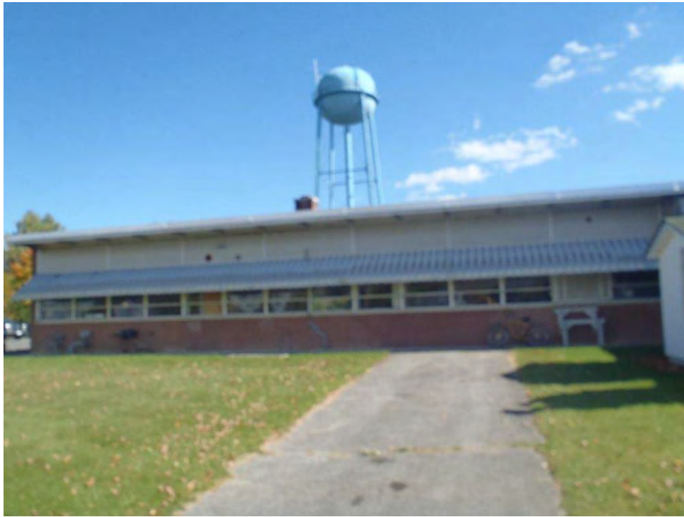
Photo 31: Warehouse building facing north.
