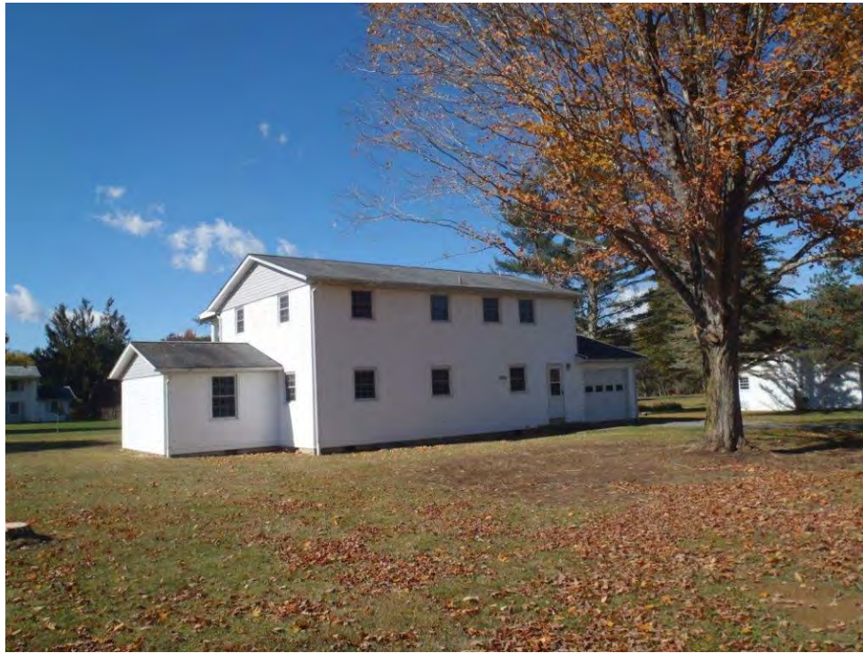
Photo 41: House #6 facing southwest.
