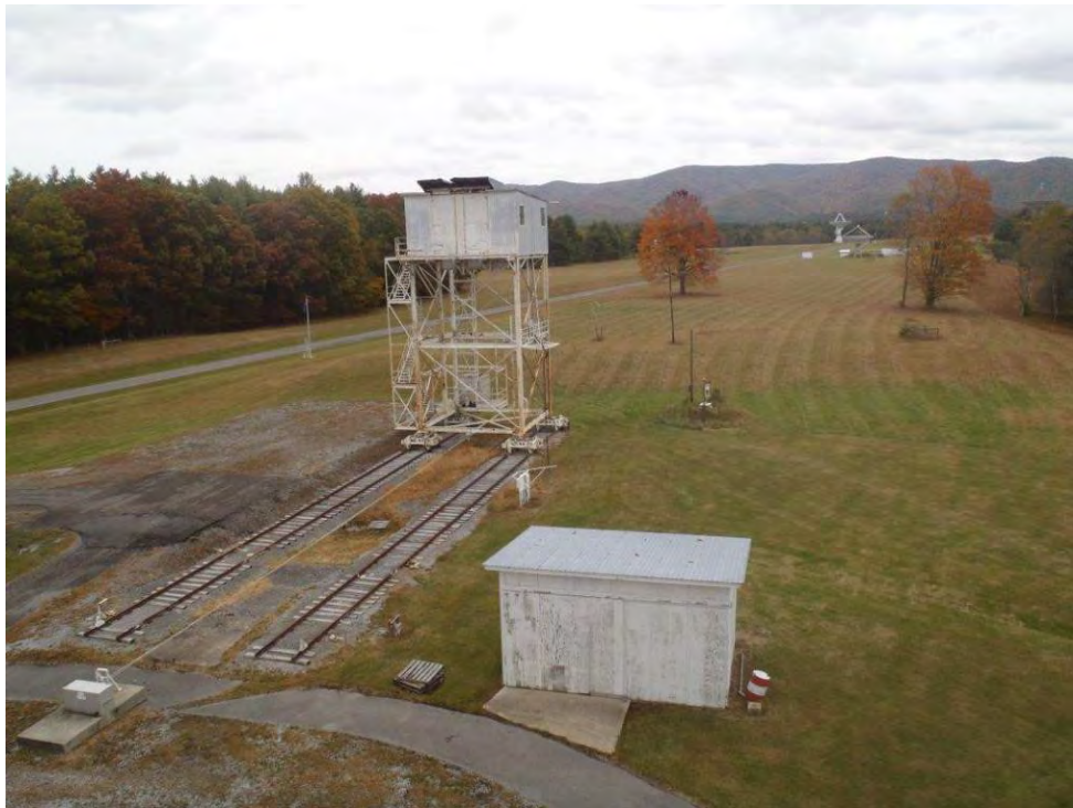
Photo 68: 140-telescope sheds facing east.
