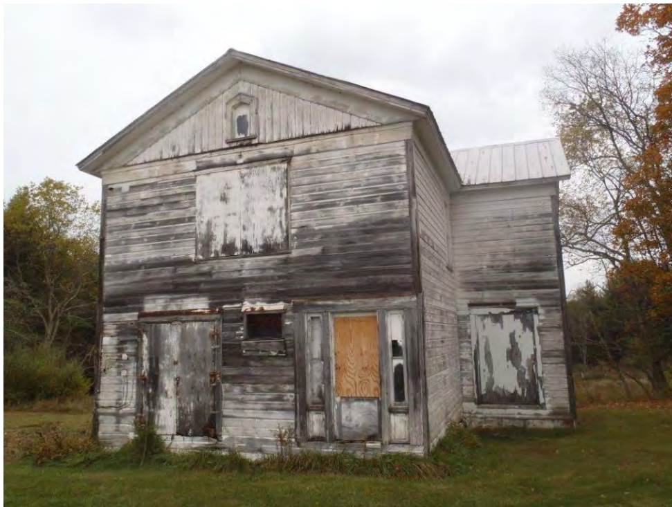
Photo 20: Beard House facing north.
