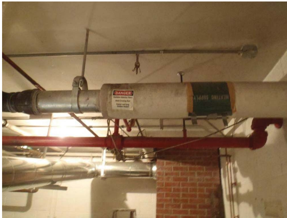
Photo 103: Encapsulated ACM at Jansky Laboratory.
