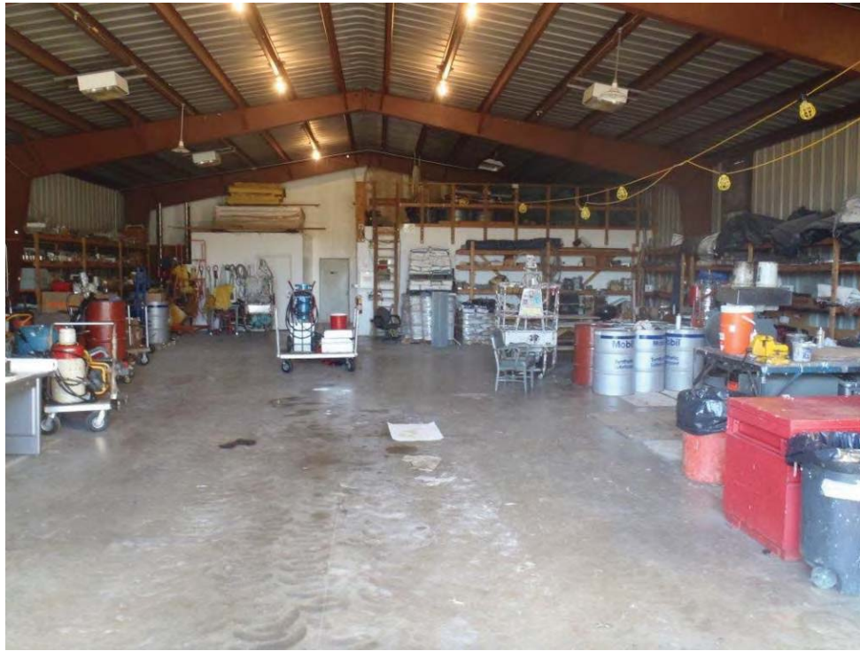
Photo 17: Inside GBT storage building facing west.
