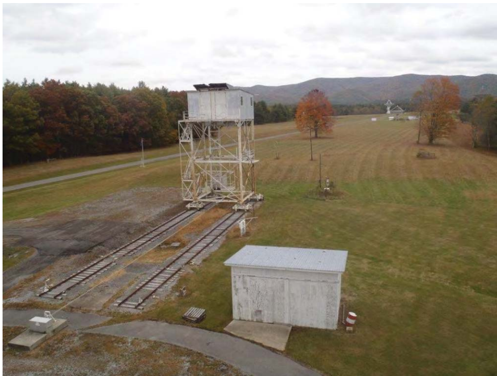
Photo 68: 140-telescope sheds facing east.
