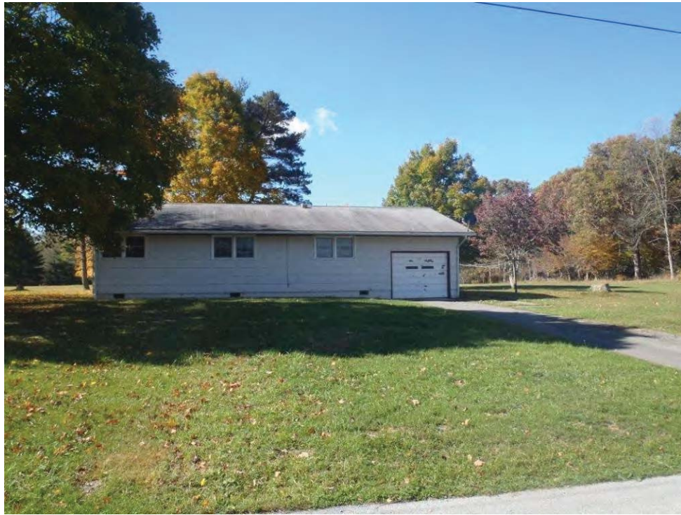
Photo 45: House #10 facing southwest.
