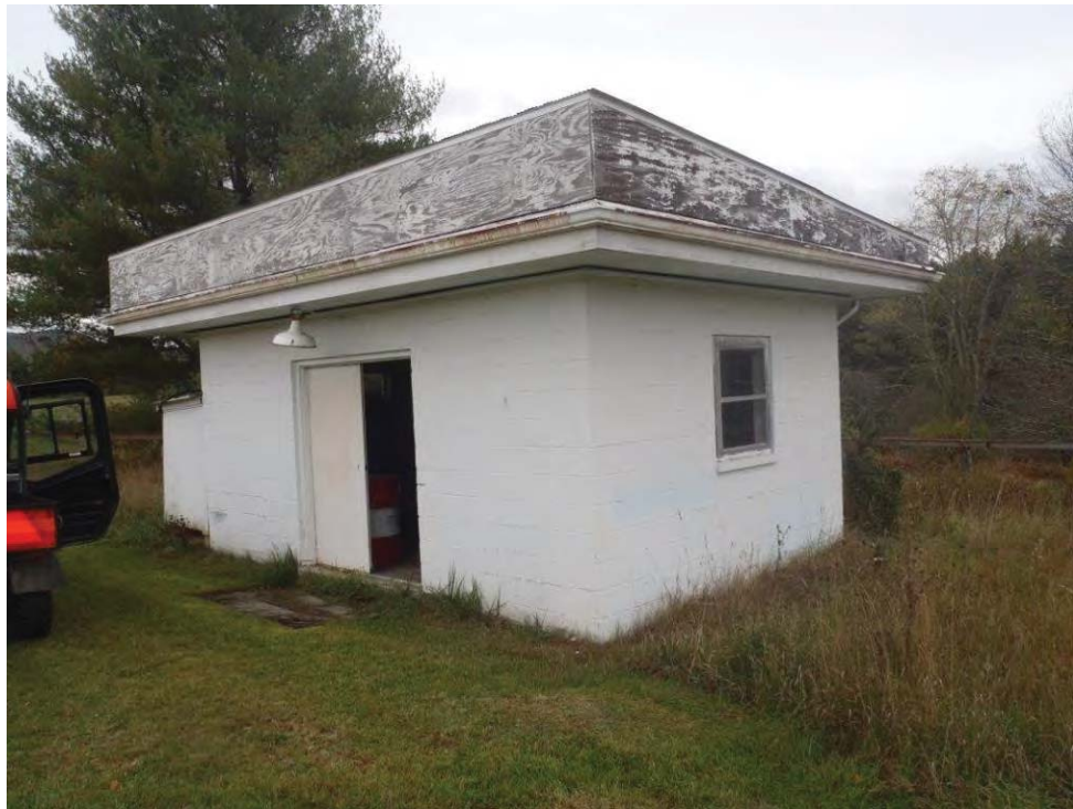
Photo 66: Sheds southwest of 85-1.
