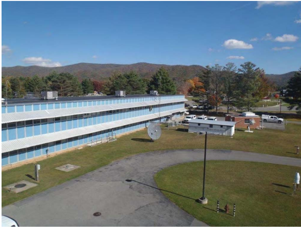
Photo 27: Jansky Laboratory facing northeast.
