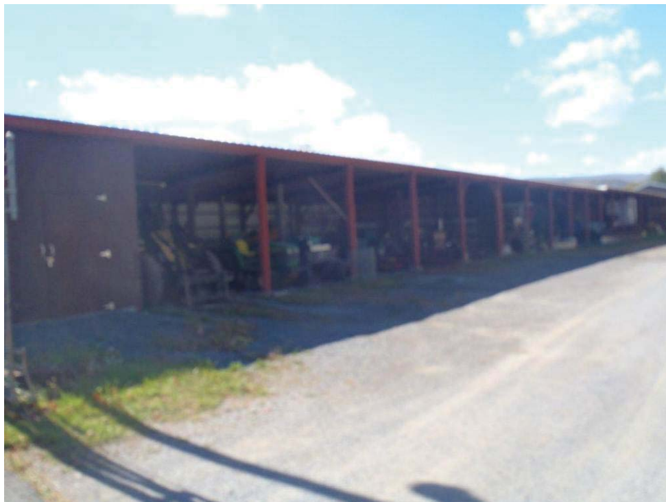
Photo 30: Covered storage at works area facing west.
