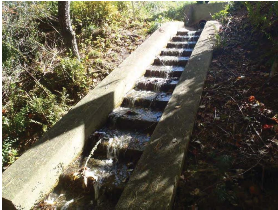
Photo 77: Outfall at wastewater treatment ponds facing south.
