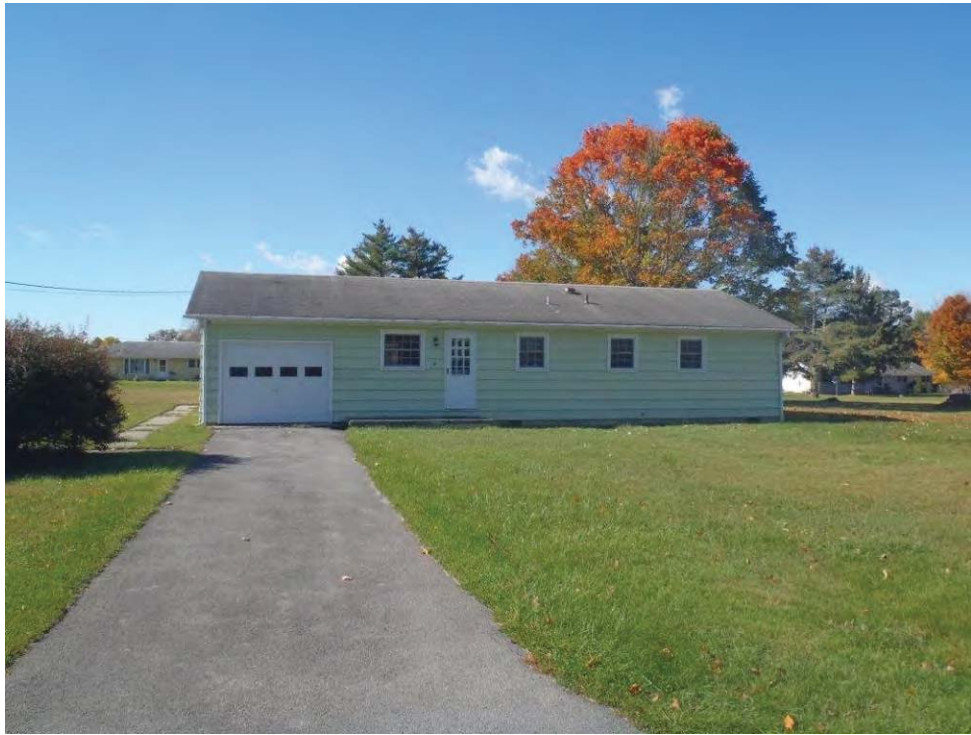
Photo 39: House # 4 facing southwest.
