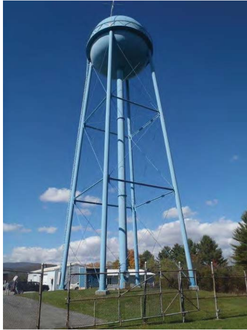
Photo 73: 100,000-gallon water tower facing northwest.
