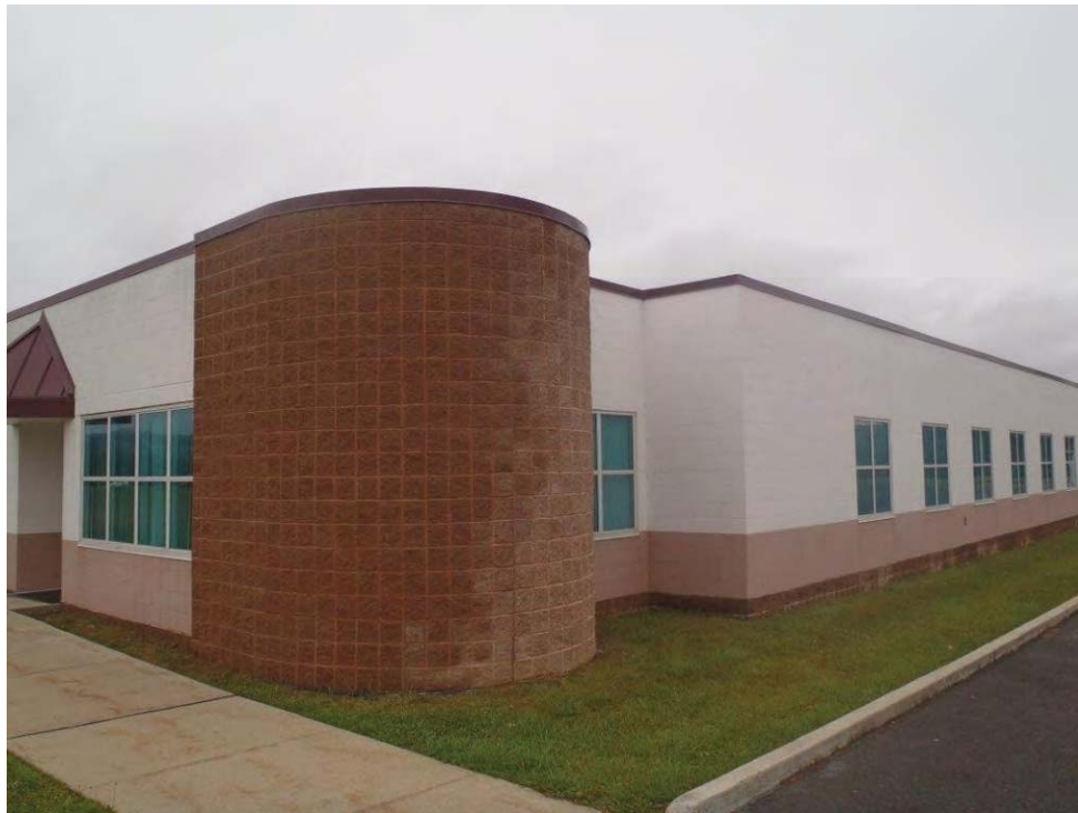
Photo 34: Bunk house facing north.
