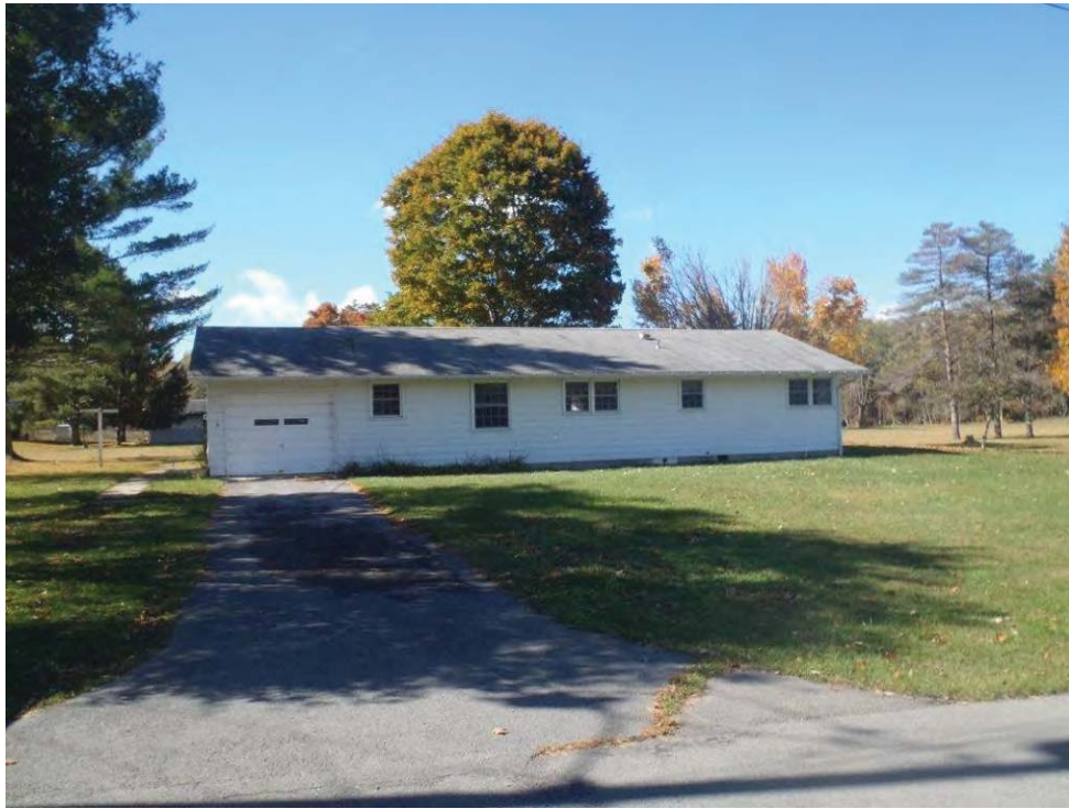
Photo 43: House #8 facing southwest.
