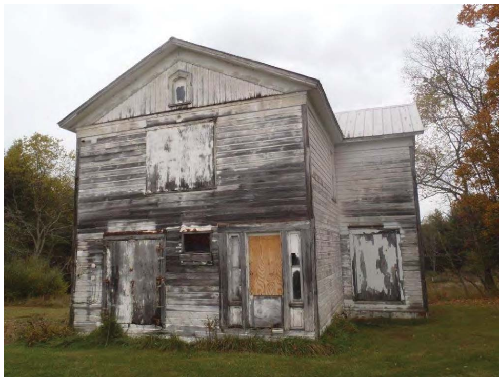
Photo 20: Beard House facing north.
