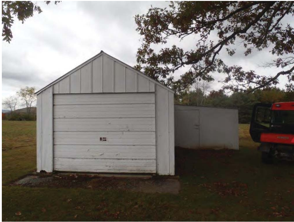
Photo 65: Sheds east of 85-1.
