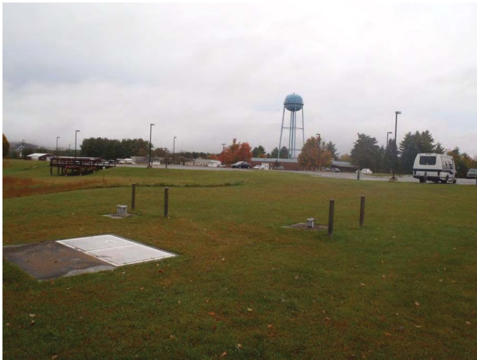
Photo 72: Drinking water wells facing north.
