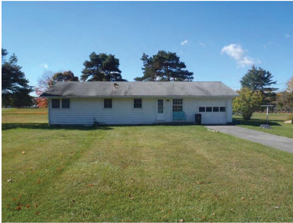
Photo 37: House #2 facing southwest.
