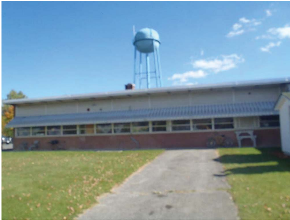
Photo 31: Warehouse building facing north.
