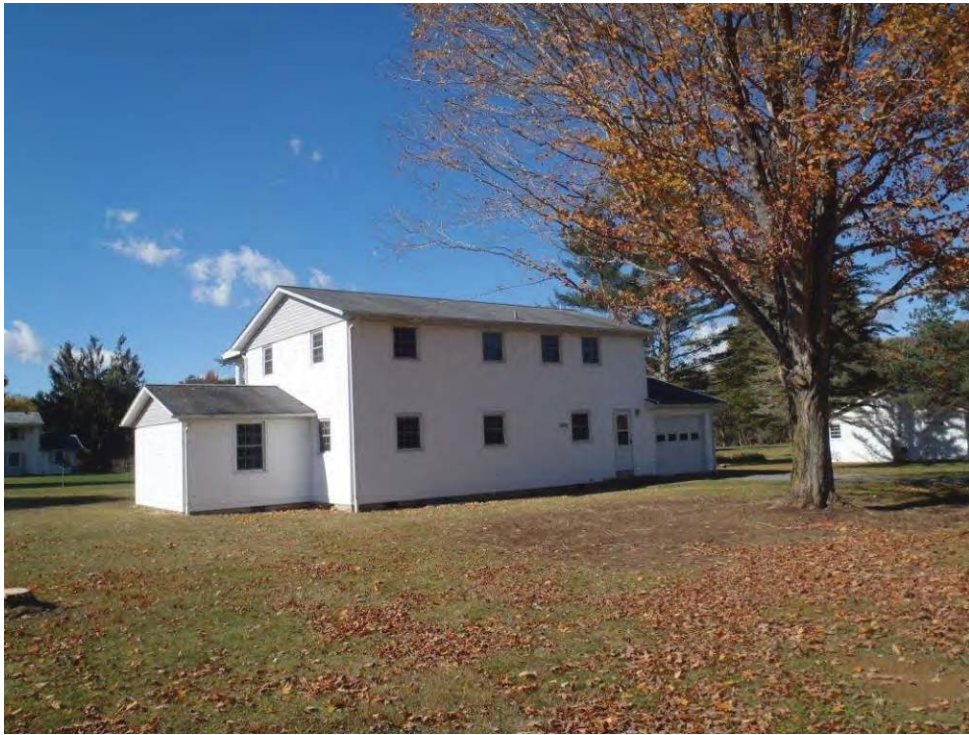
Photo 41: House #6 facing southwest.
