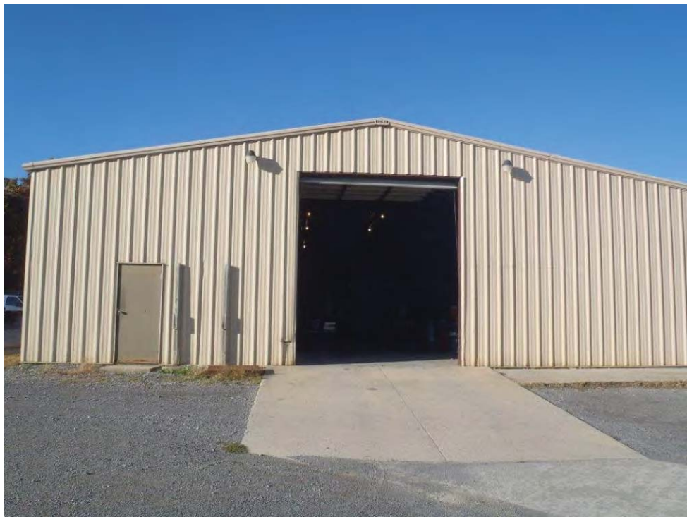
Photo 16: GBT storage building facing west.
