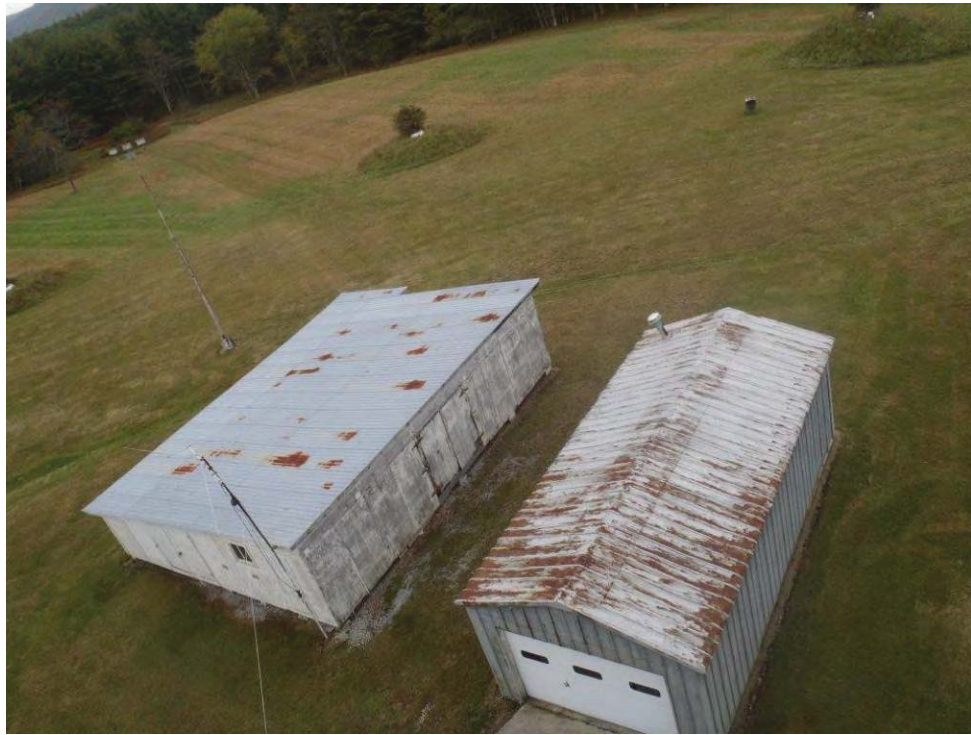
Photo 69: 140-telescope sheds facing east.
