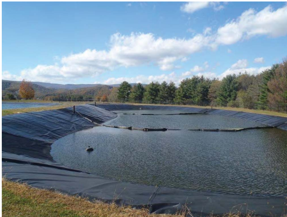
Photo 74: Wastewater treatment ponds facing west.
