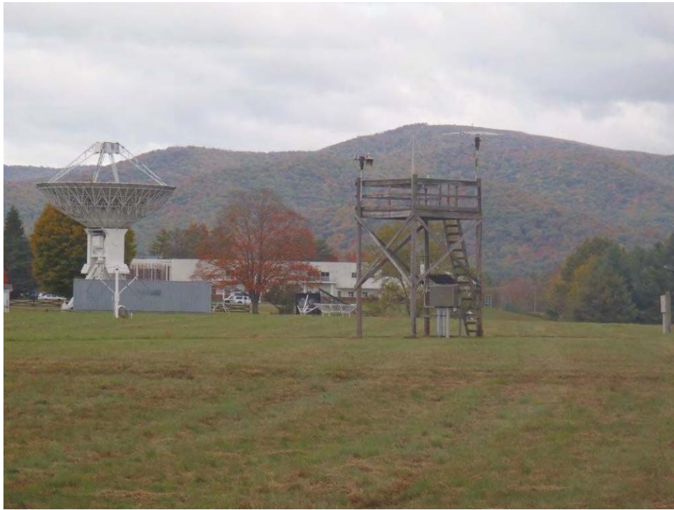
Photo 67: Weather station facing north.
