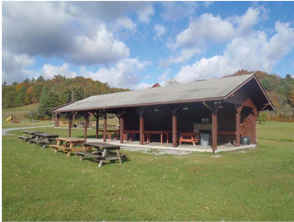
Photo 61: Pavilion facing north.
