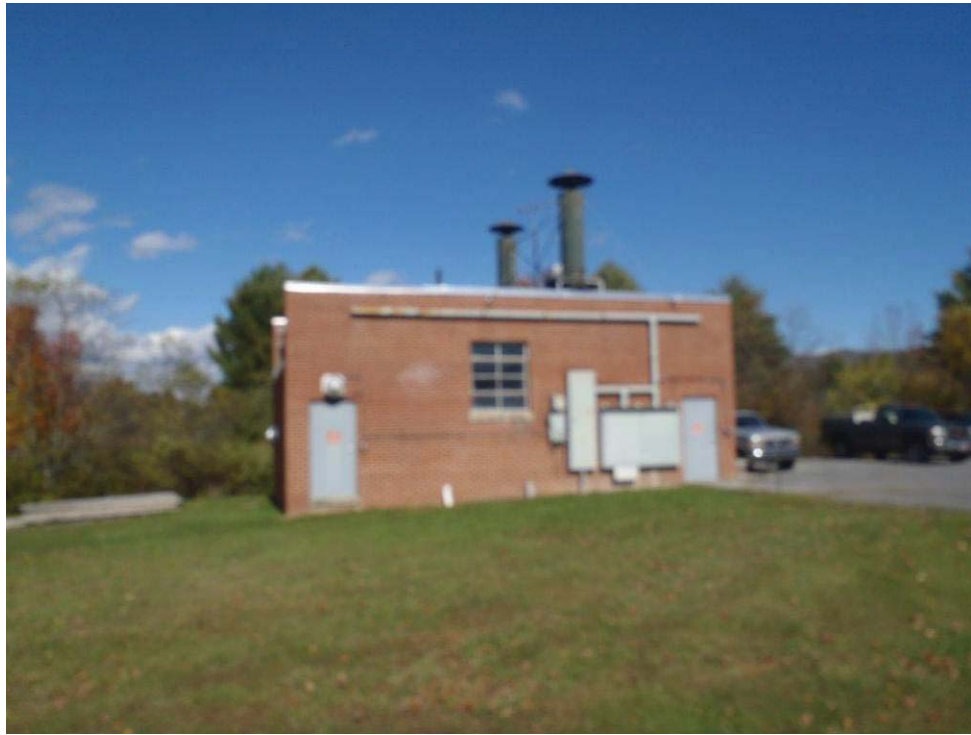
Photo 33: Paint booth facing north.
