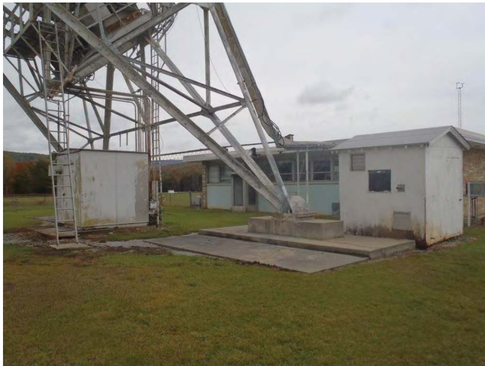
Photo 22: Shed at 85-1 facing northeast.
