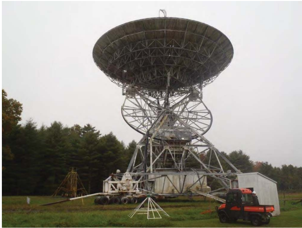
Photo 9: 85-3 interferometer facing south.
