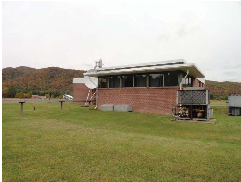
Photo 11: Former interferometer control building facing north.
