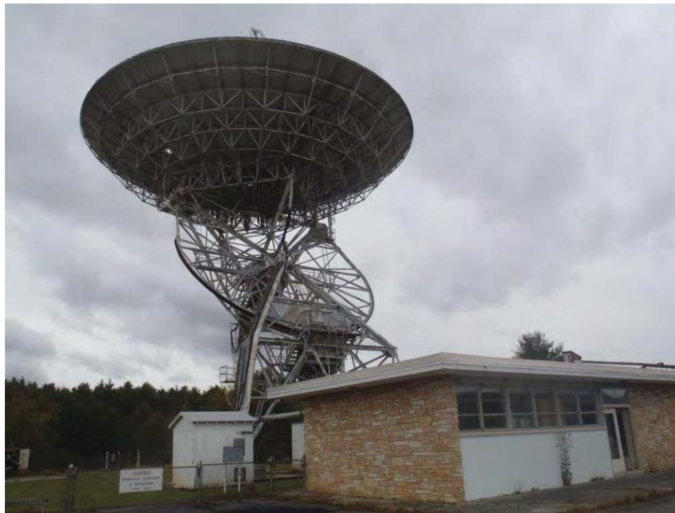
Photo 7: 85-1 interferometer facing south.
