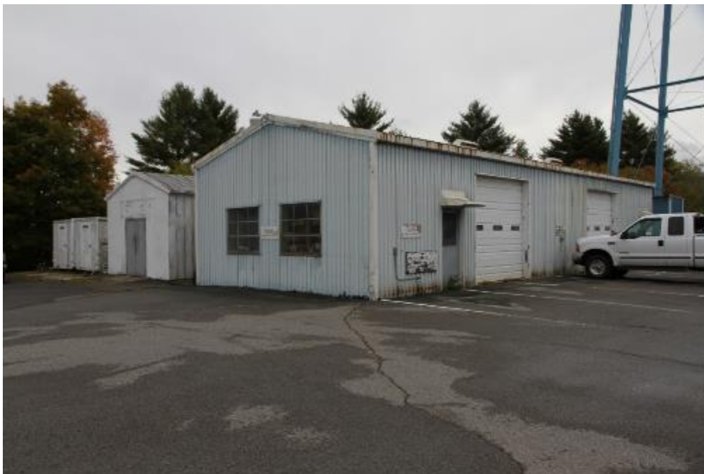
FIGURE 3.3-6 Sample Utilitarian Buildings, Mechanics Building and Water Tower (2014).
