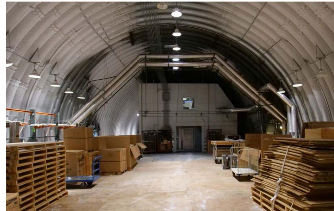
WAREHOUSING IN THE LOGISTICS ARCH. The logistics arch and heated warehouse building have a structural steel and plywood floor to allow the forklift use and pallet storage; the floor is beginning to dome. Source: NSF, Josiah Horneman, 2021.
