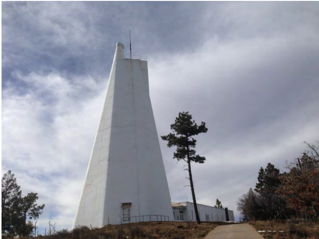
Photo 47: Dunn Solar Telescope facing northwest
