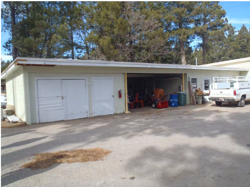
Photo 26: Maintenance equipment storage and office facing northwest
