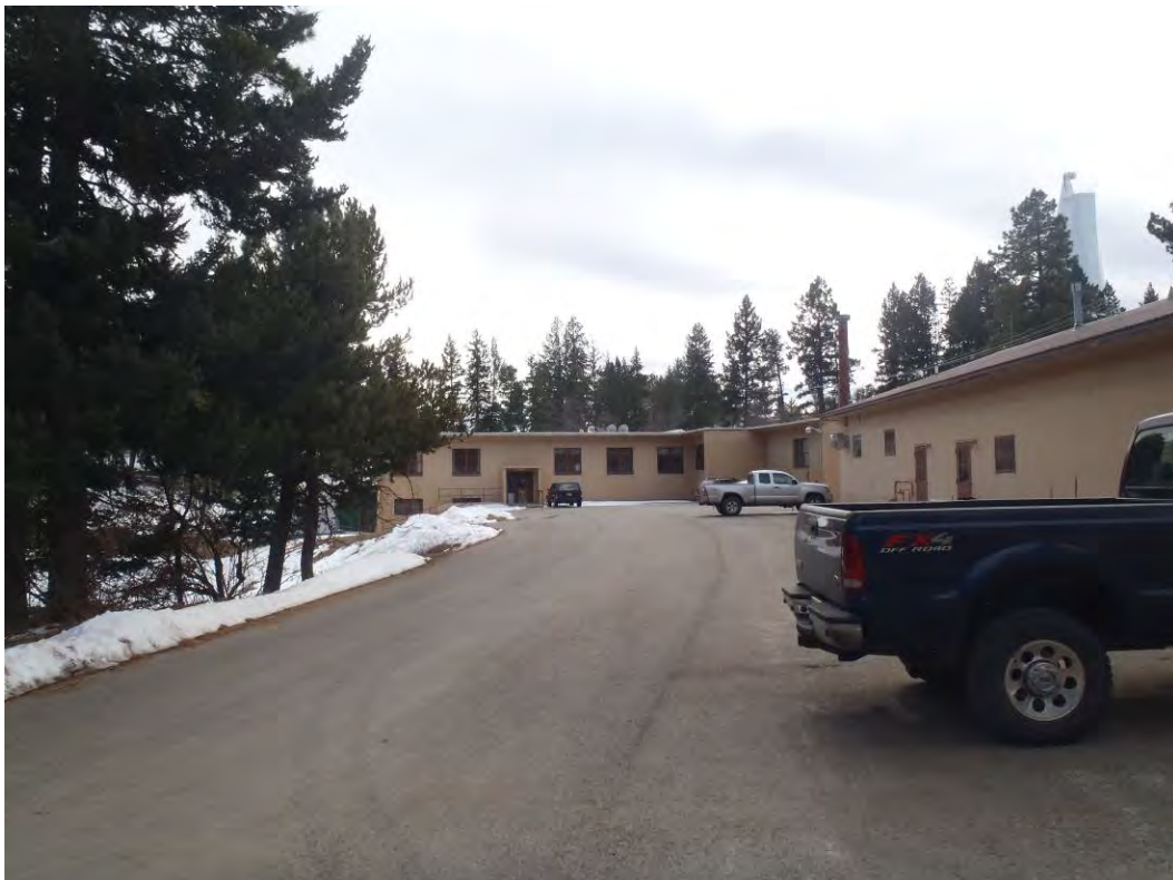
Photo 34: Main laboratory (far back) and maintenance shop (right) facing south
