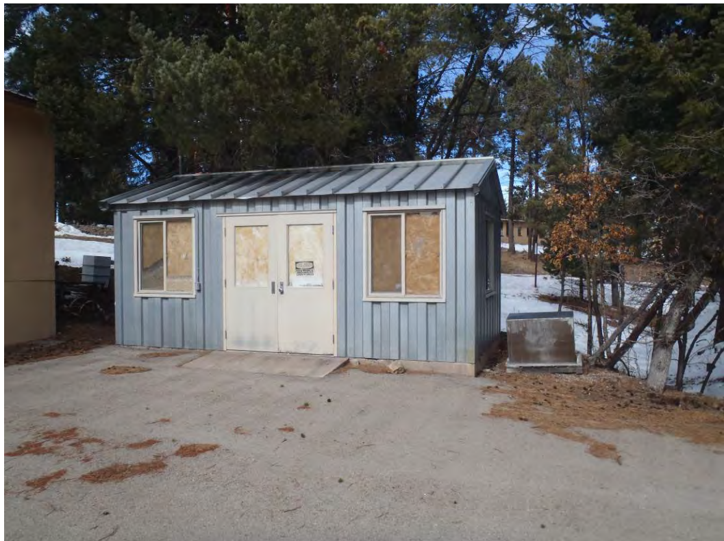
Photo 30: Paint booth facing north
