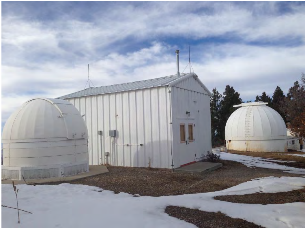
Photo 53: Former ISOON telescope building facing west
