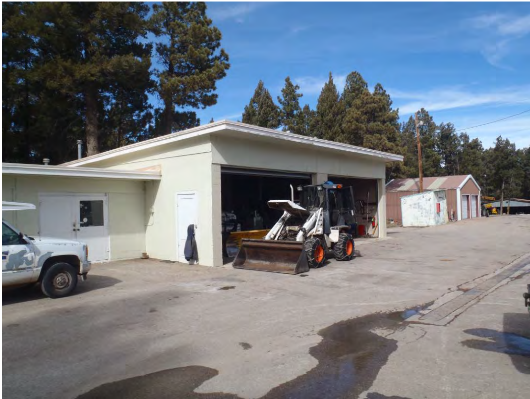
Photo 27: Maintenance garage facing northwest
