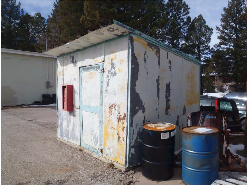
Photo 25: Former hazardous waste shed (empty)
