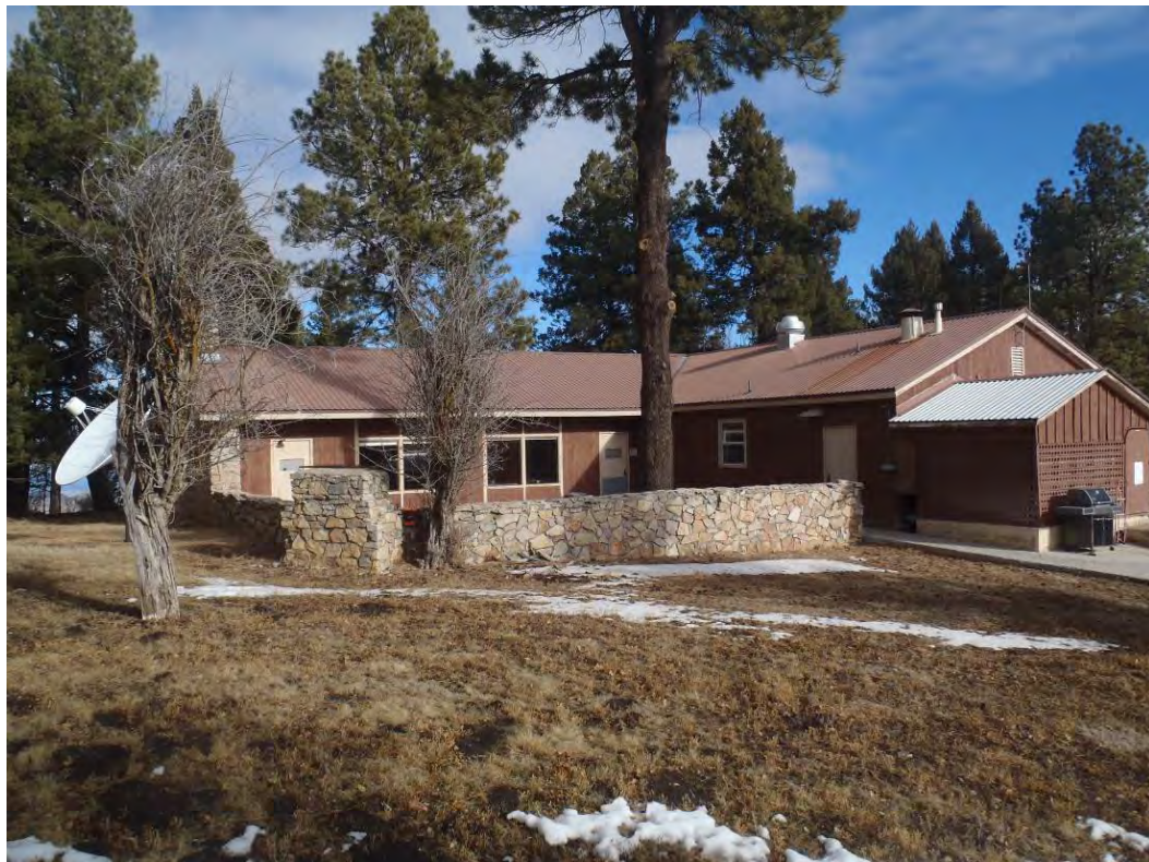
Photo 60: Administration and café building facing north
