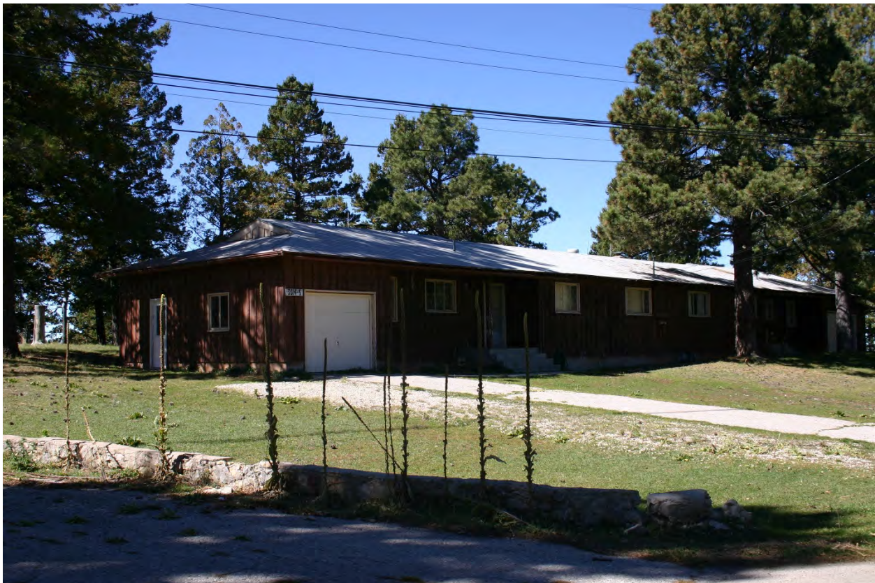
Photo 3. Building 3014, Redwood Family Housing Duplex
