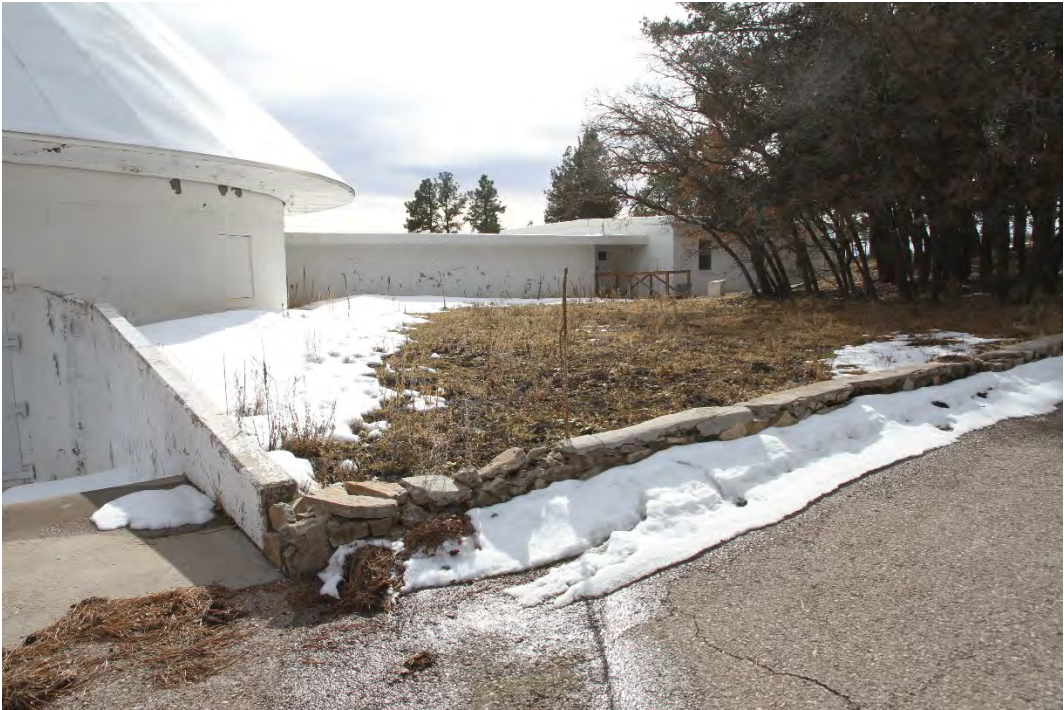
Photo 10. Stone wall adjacent to the John W. Evans Solar Facility
