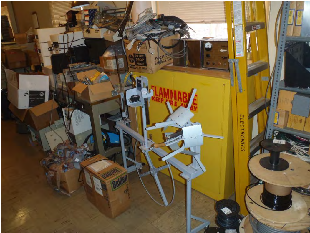
Photo 37: Flammable locker inside main lab
