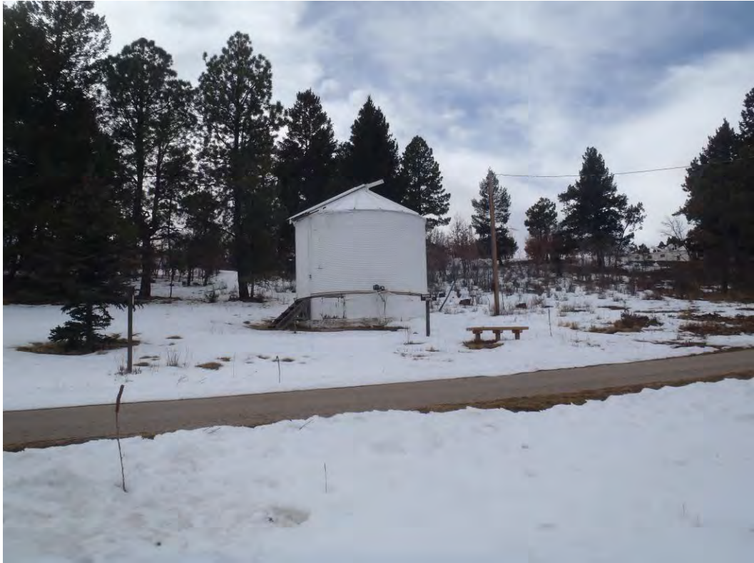
Photo 45: Grain Bin Telescope facing west
