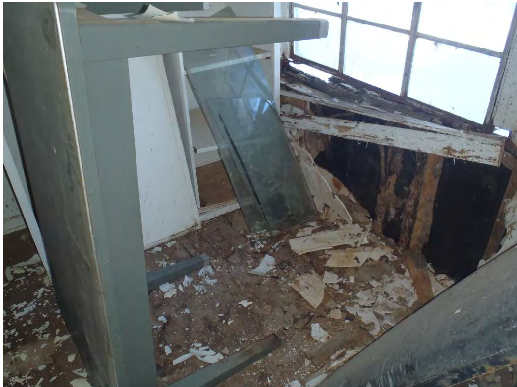
Photo 70: Inside Quonset hut near residential area
