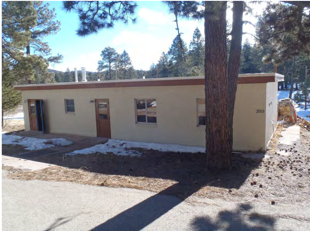
Photo 71: Laundry building facing southeast
