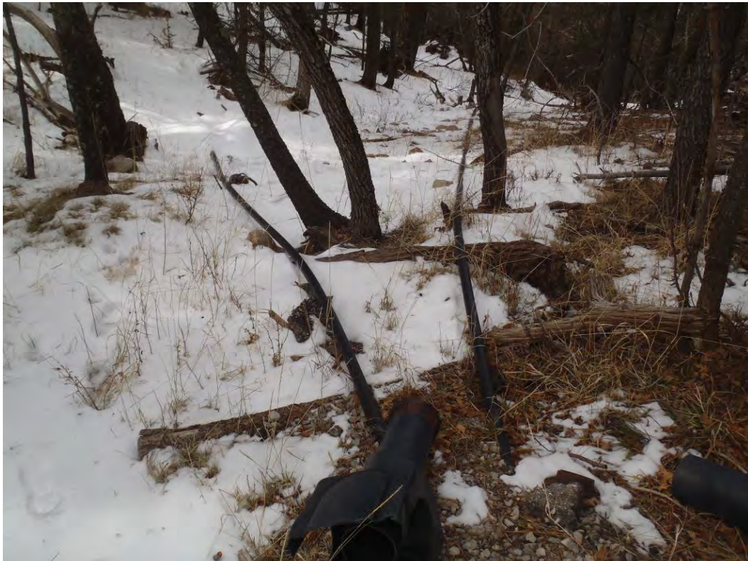
Photo 7: Wastewater discharge perforated piping facing west
