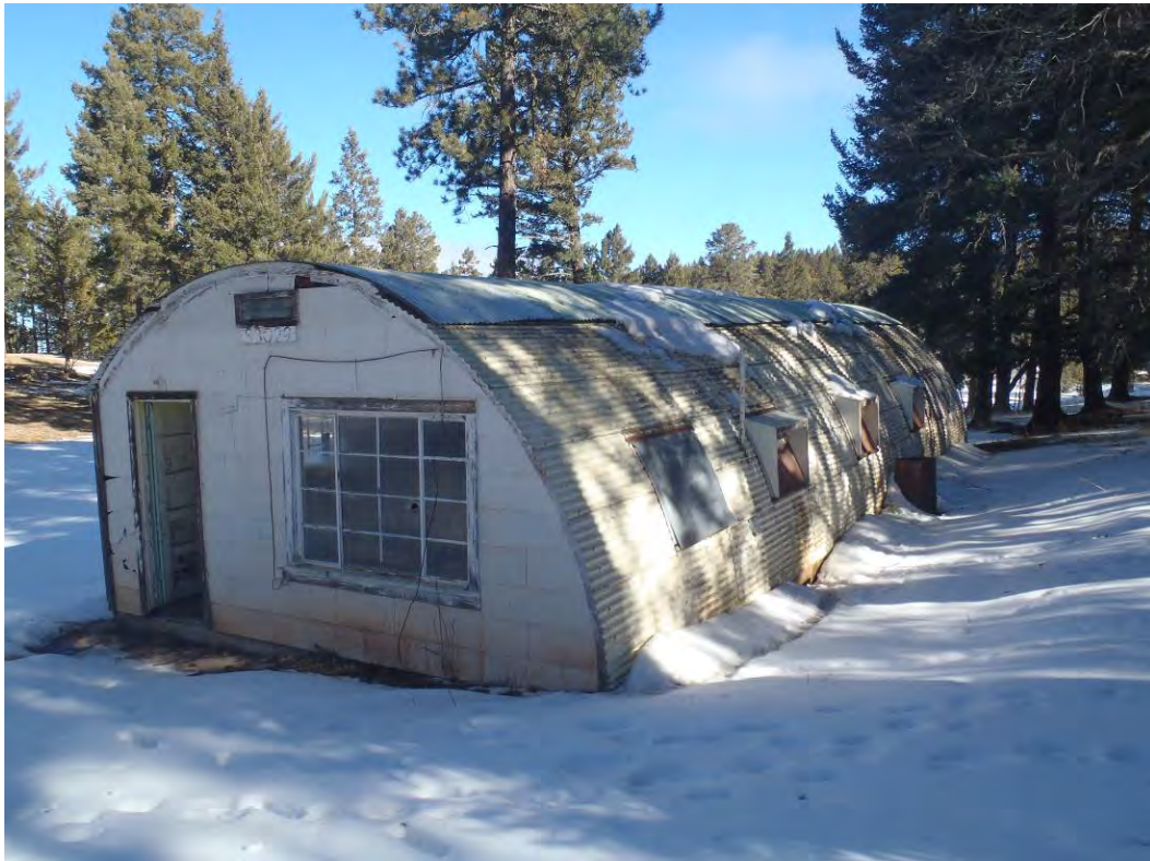
Photo 69: Quonset hut near housing area facing north
