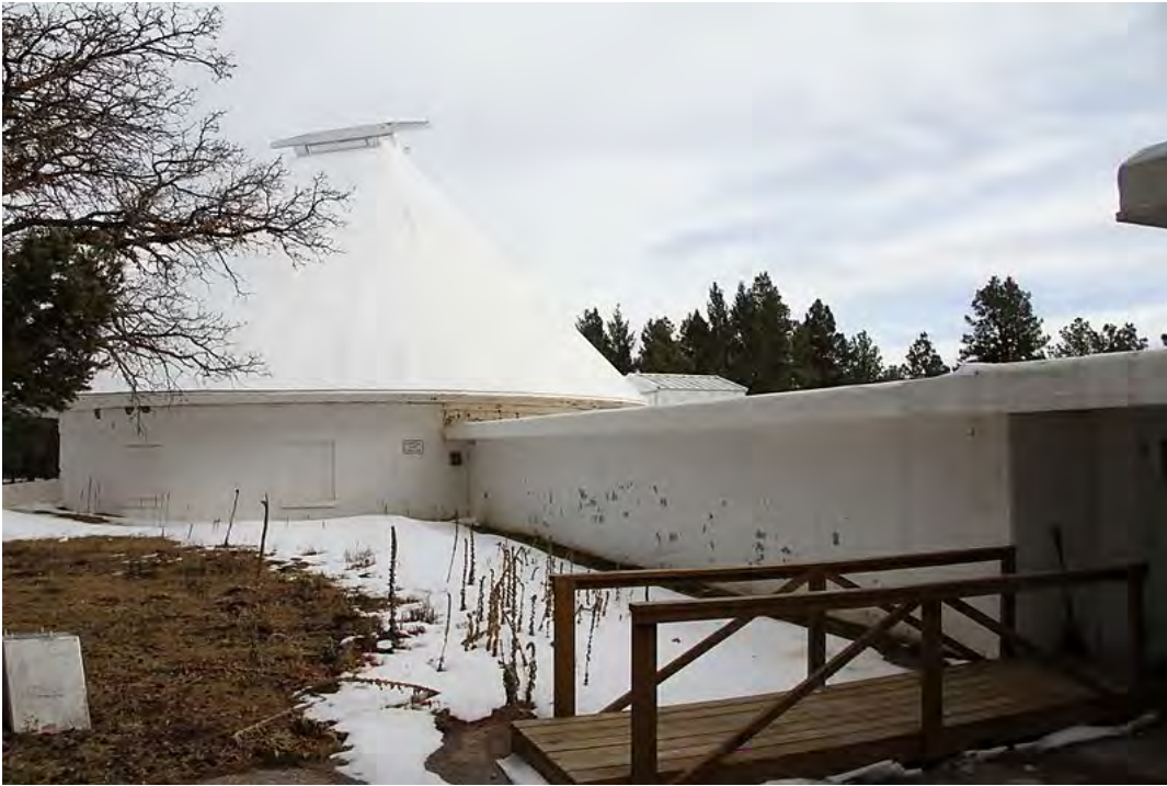
Photo 2. The John W. Evans Solar Facility (formerly the Big Dome)
