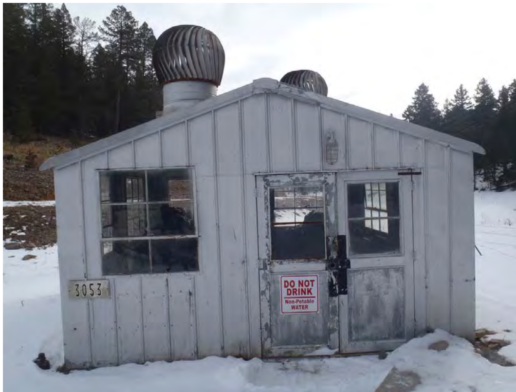
Photo 4: Wastewater pump house facing north
