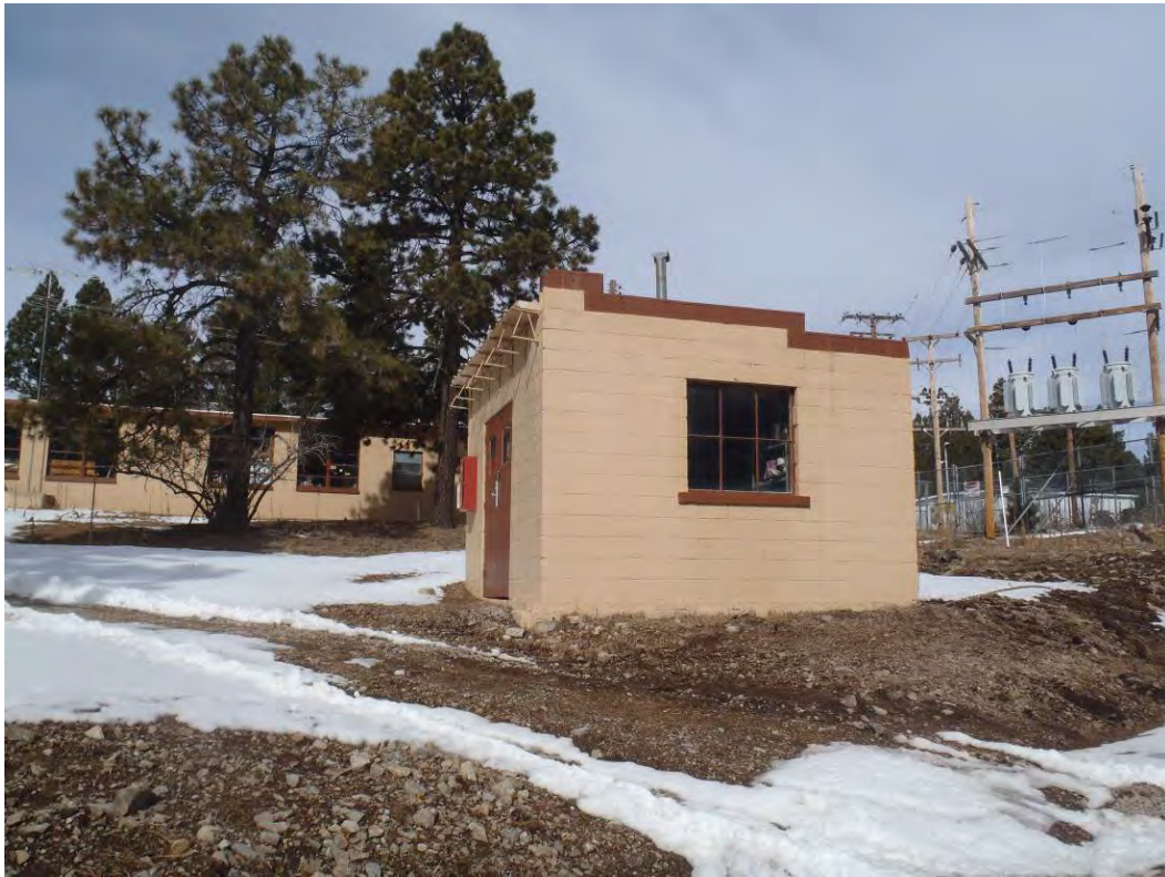
Photo 15: Paint storage building facing north
