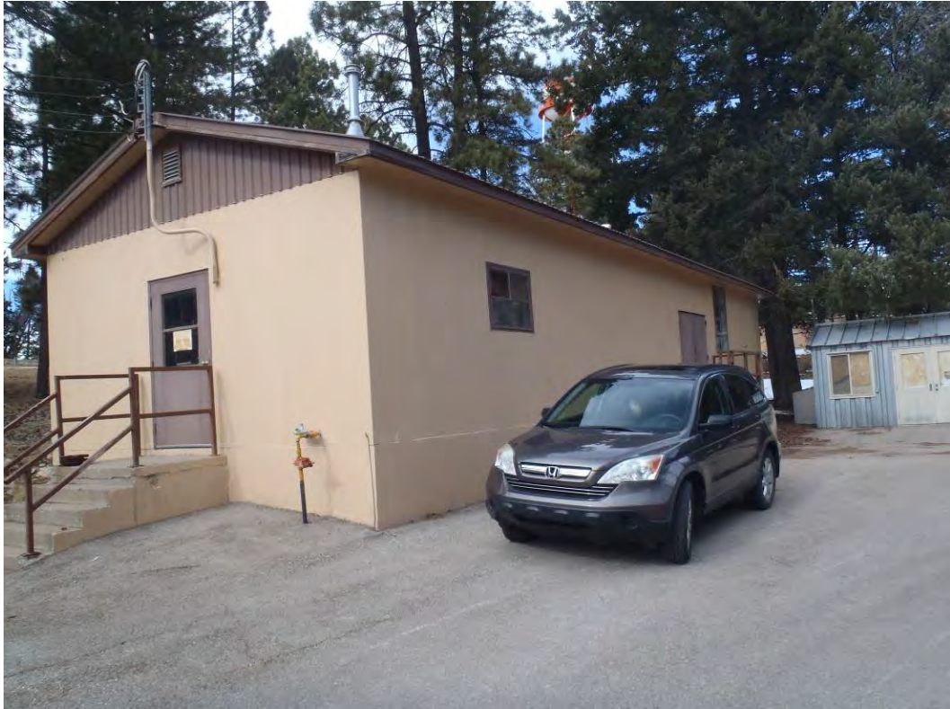
Photo 29: Library and welding shop building facing northwest
