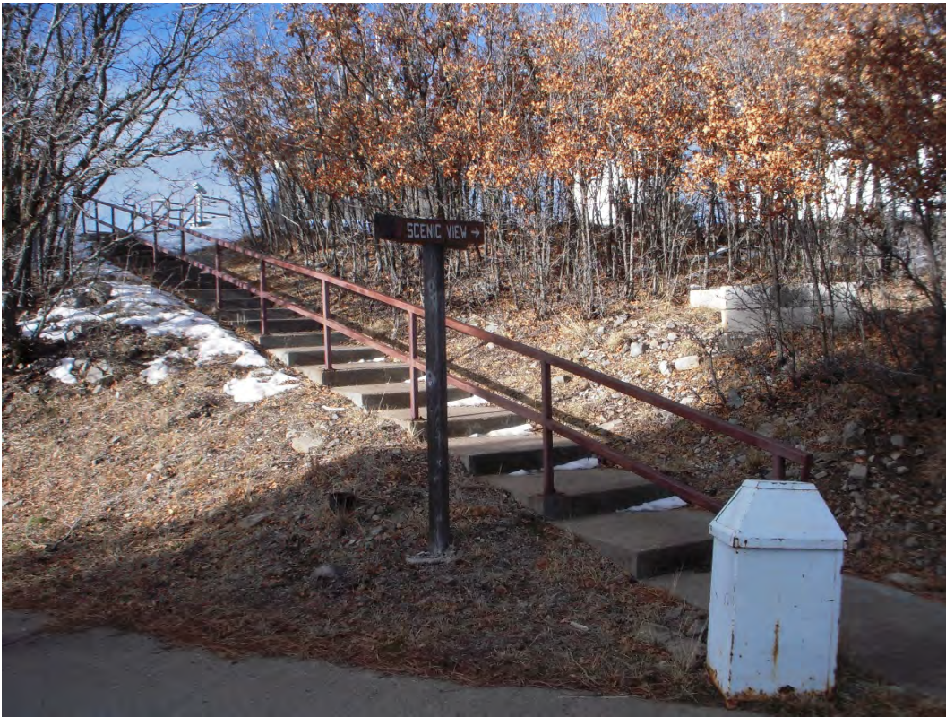
Photo 11. Outdoor stairwell near the DST
