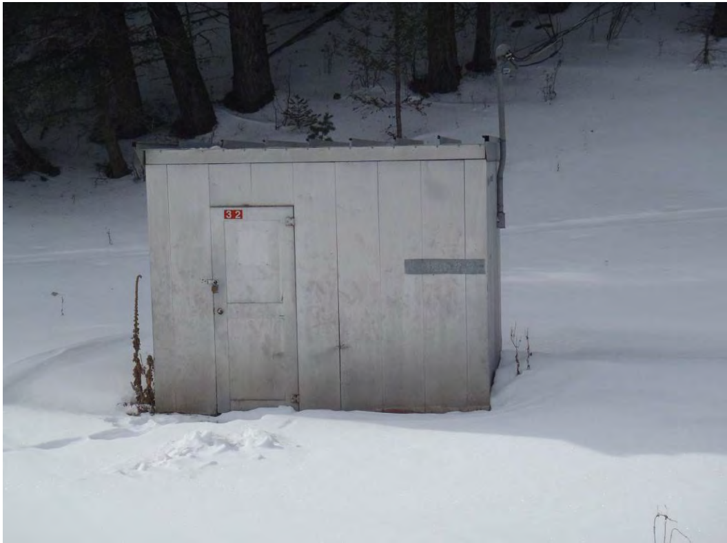
Photo 2: Water well #2 facing south
