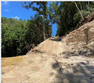
Tower 4 temporary access road
