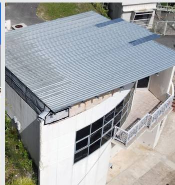
5 Learning Center temporary roof
