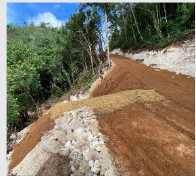
Erosion control measures after Tower 4 pieces recovered
