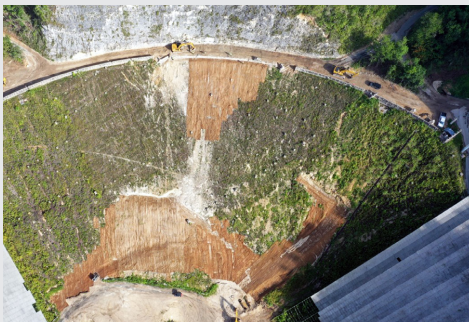
2 Rim wall repairs and erosion control measures
