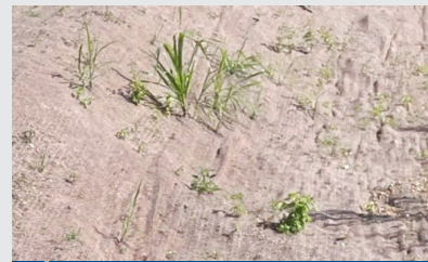
3 Coconut matting for site stabilization
