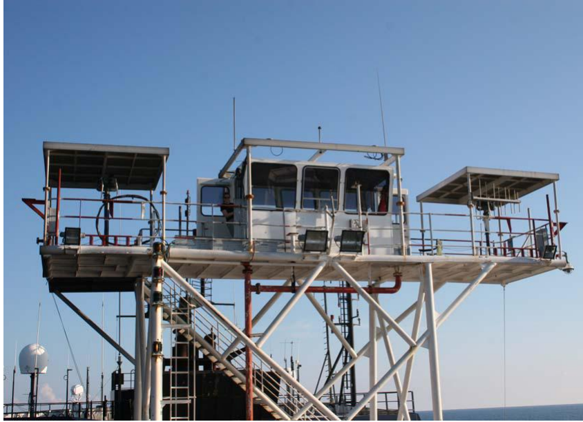
Figure 2. Protected Species Observer observation tower with mounted big-eye binoculars.
