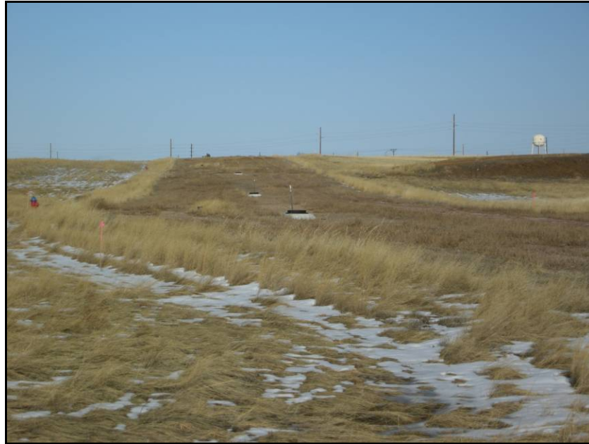
Figure 4-2. Sanitary Sewer Manholes on McKinney Drive near Proposed NWSC Site
