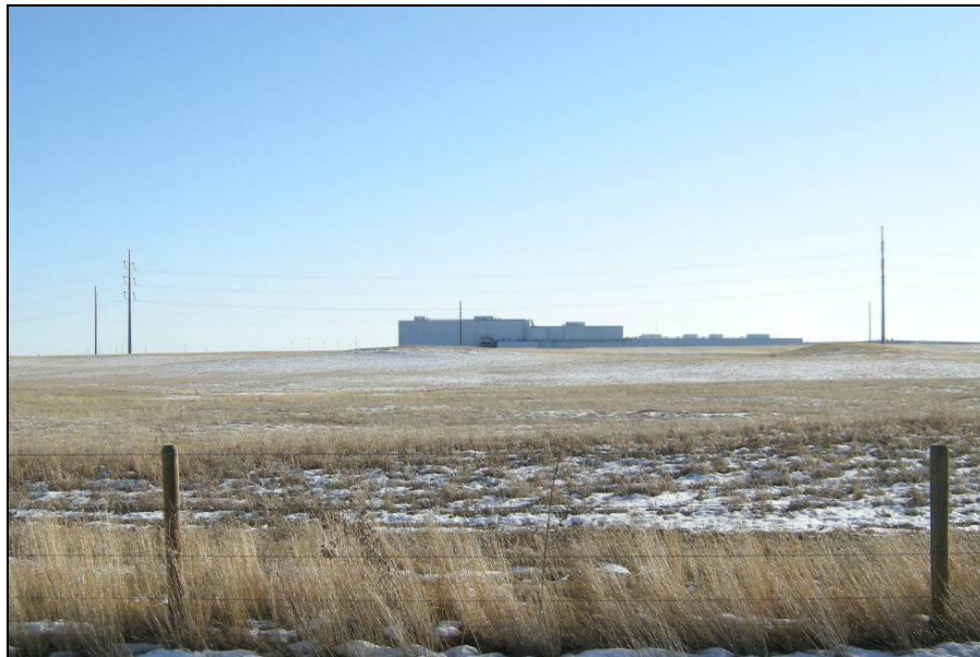
Figure 3-10. View of NWSC Site from Happy Jack Road with Power Lines and Walmart Distribution Center in Distance
